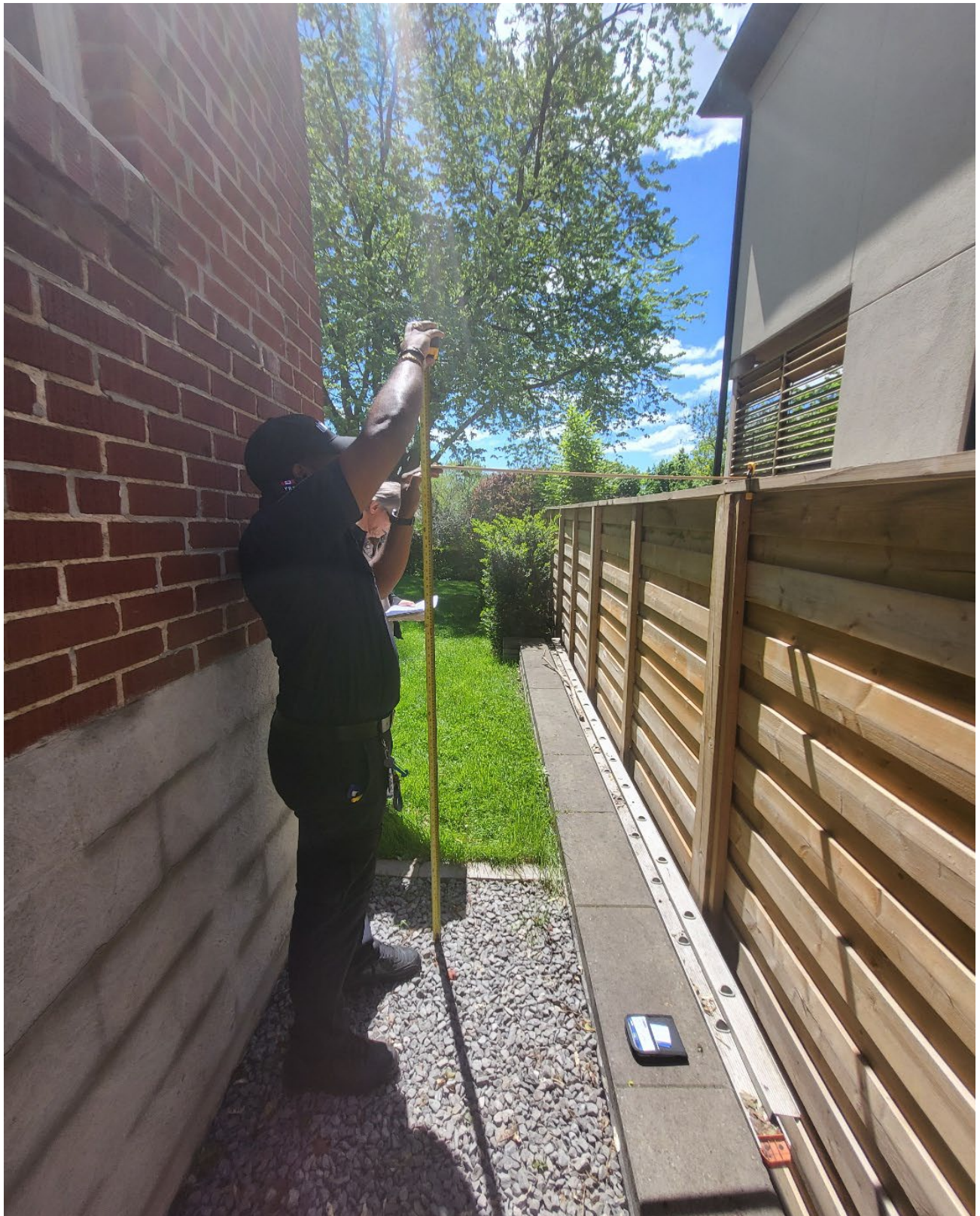
Attachment 7: Rear fence – eastern lot line fence (Panel #2) – from 63 Mayfield Avenue.
