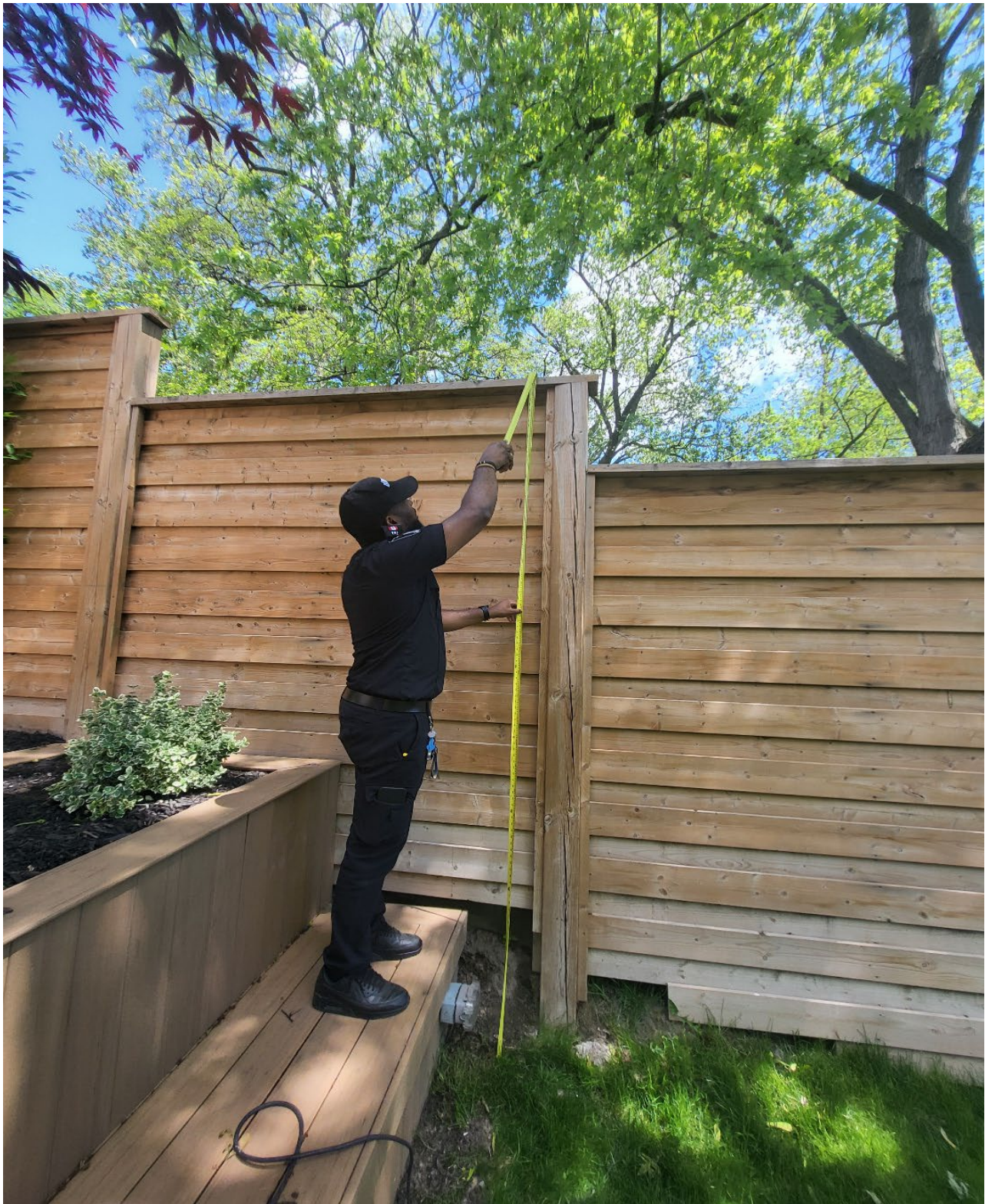
Attachment 9: Rear fence – eastern lot line fence (Panel #7) – from 65 Mayfield Avenue.
