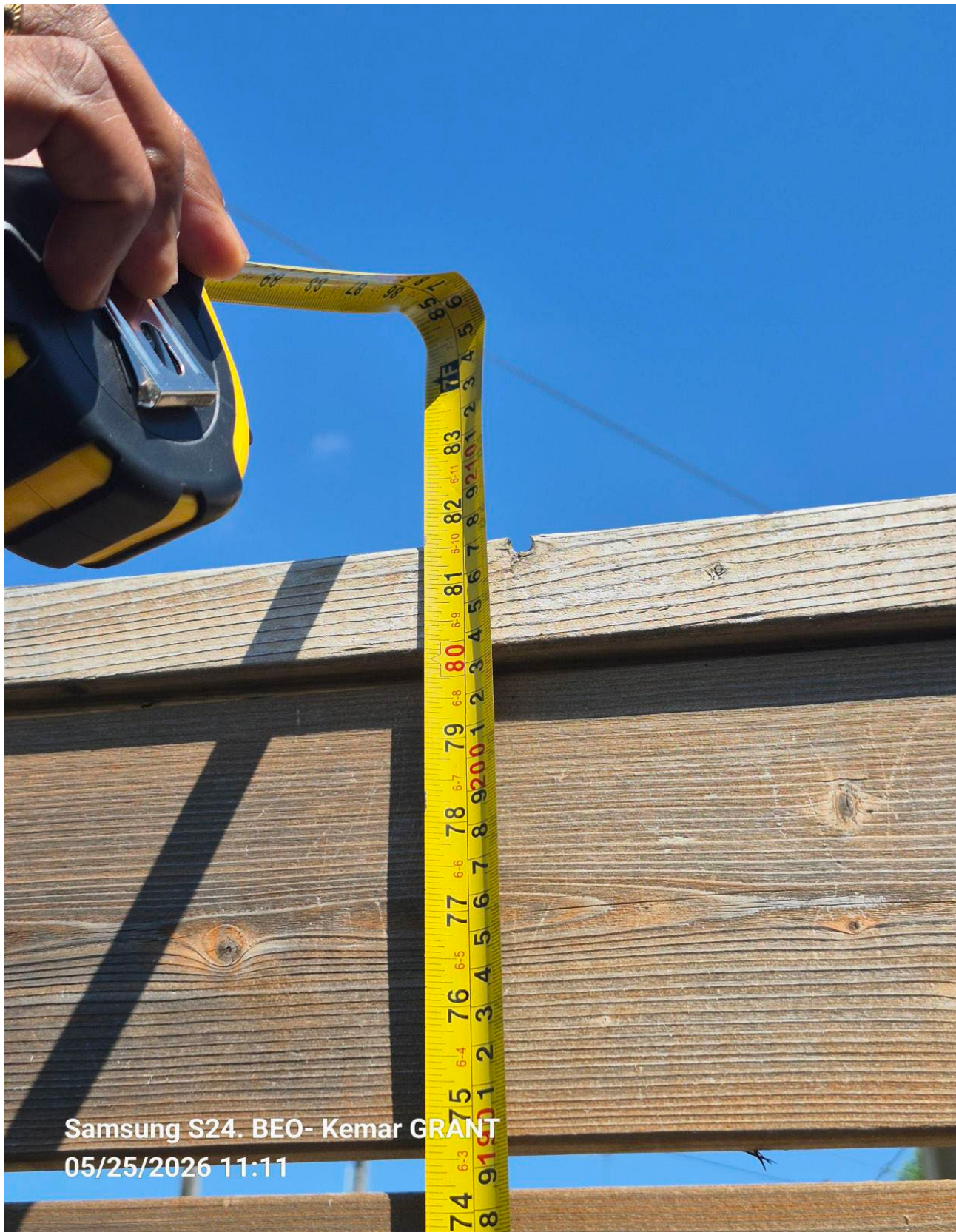
Attachment 14: Rear yard- Southern property line fence panel zoomed measurmeant
