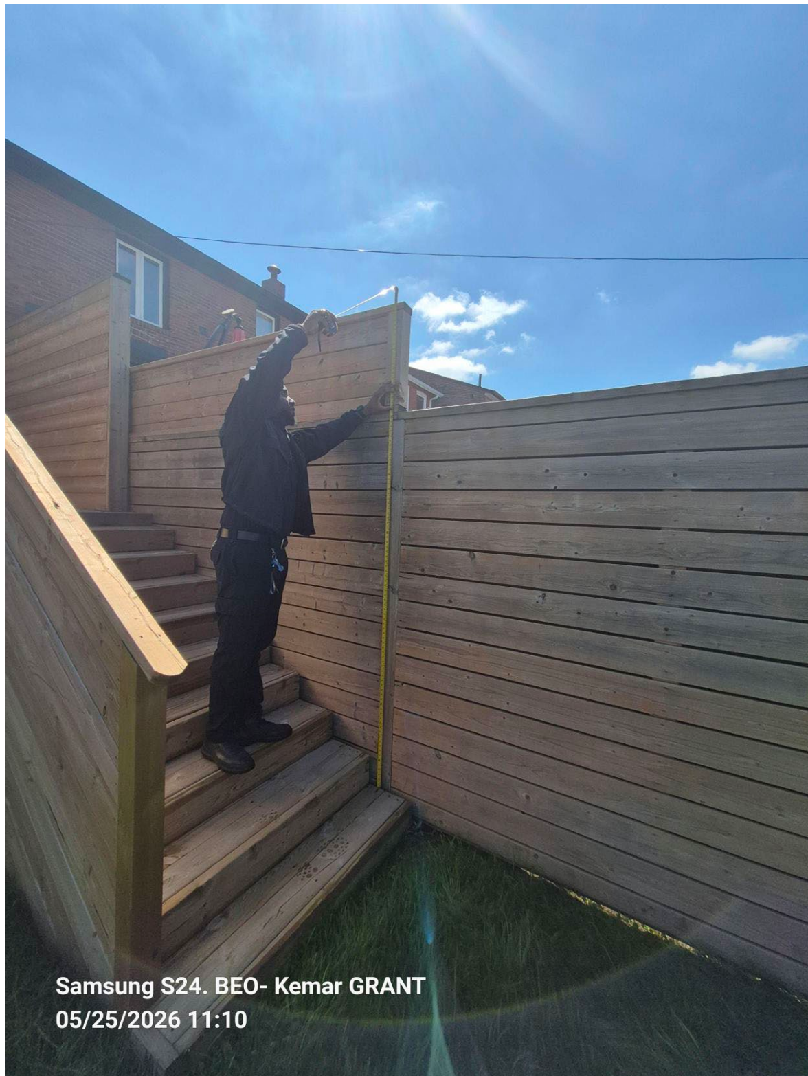
Attachment 5: Rear fence – Overview of rear yard- Eastern property line 1 st fence panel
