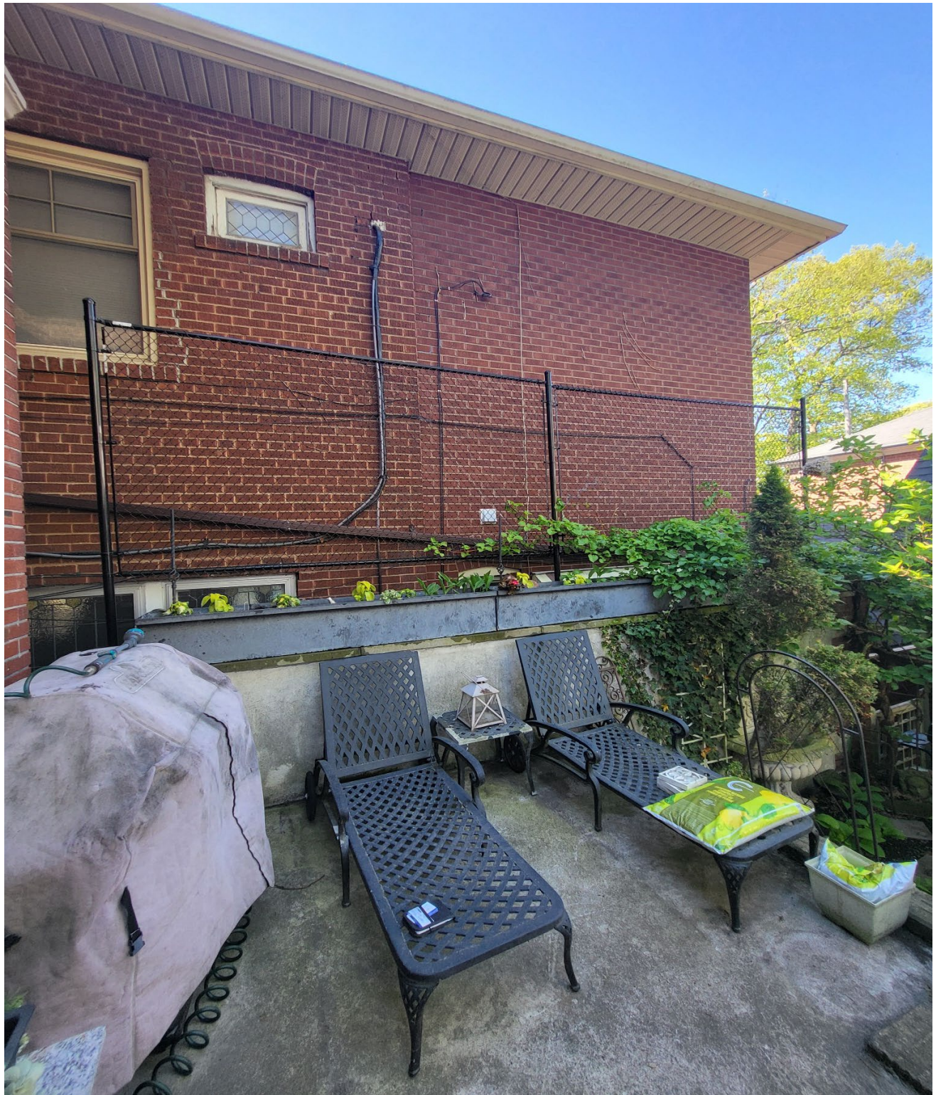
Attachment 3: Overview of Southern lot line fence
