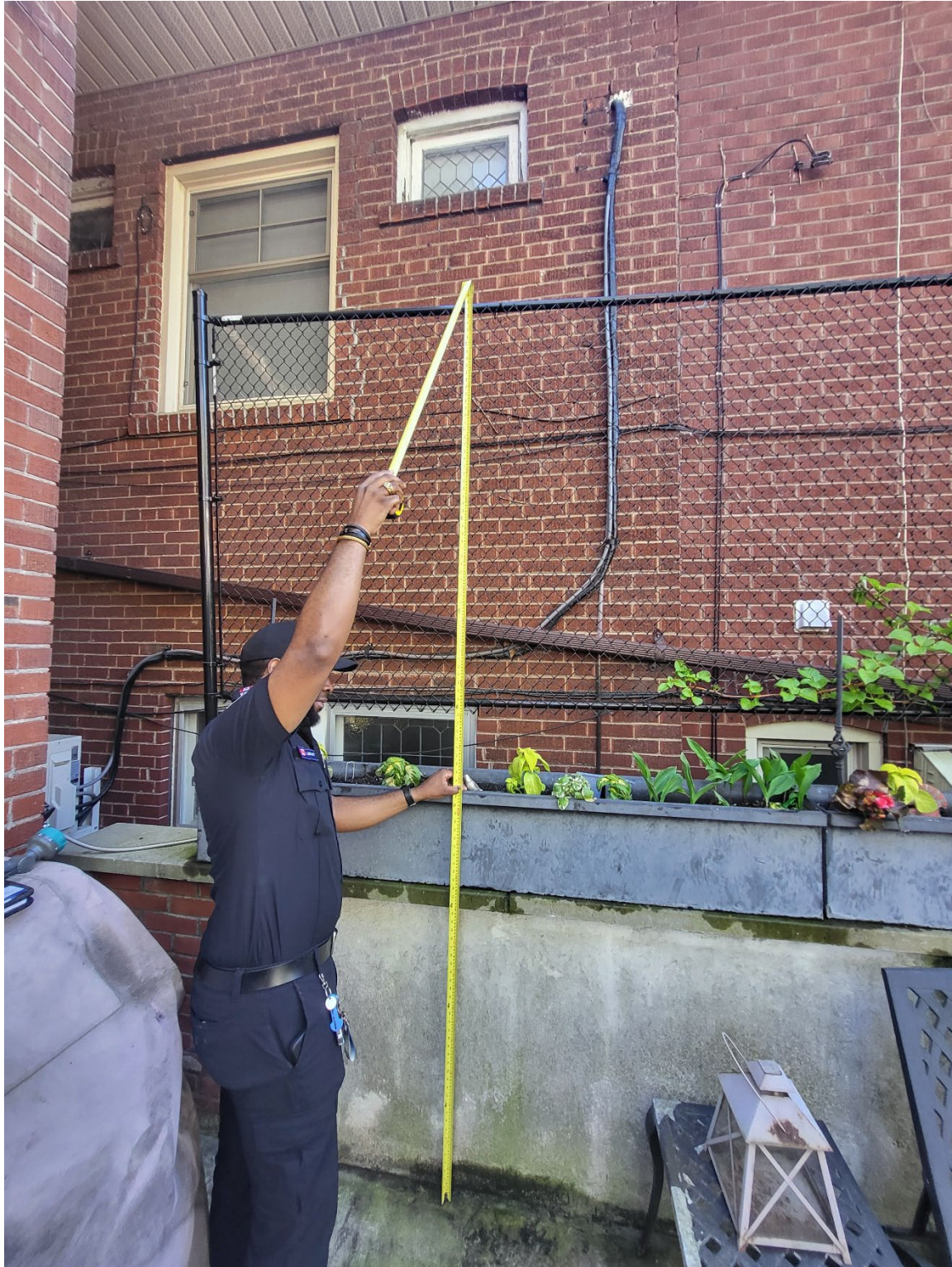
Attachment 4: Rear fence Southern lot line first section of fence
