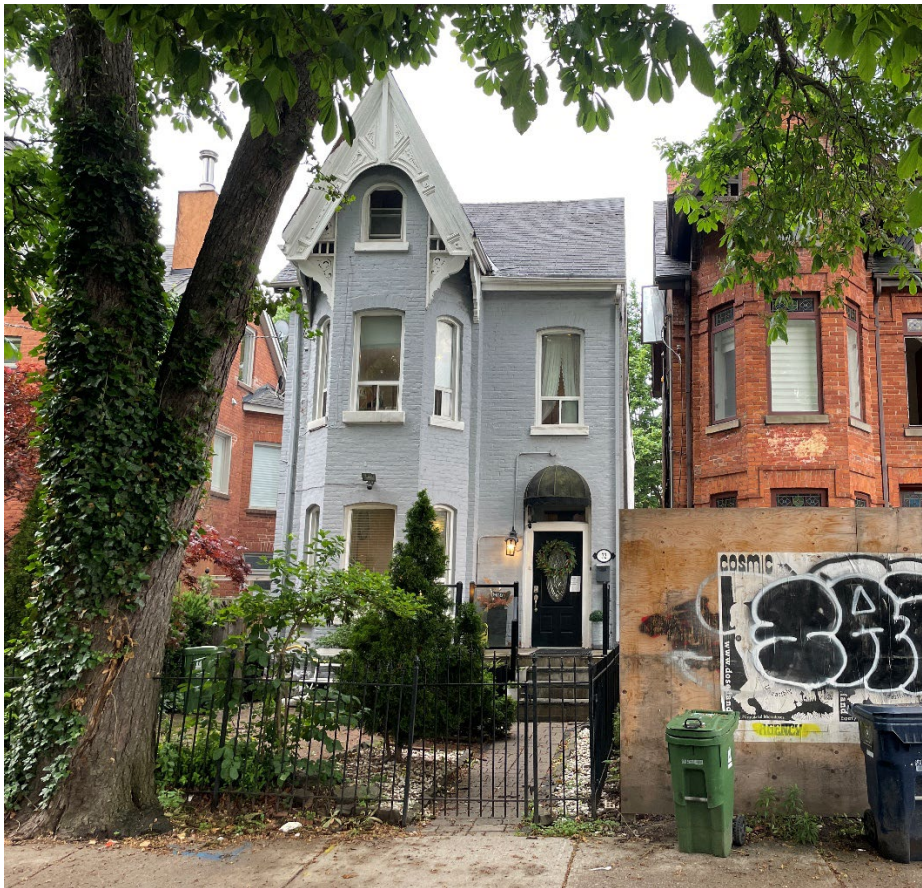
72 Henry Street, east elevation (Heritage Planning, 2026).
