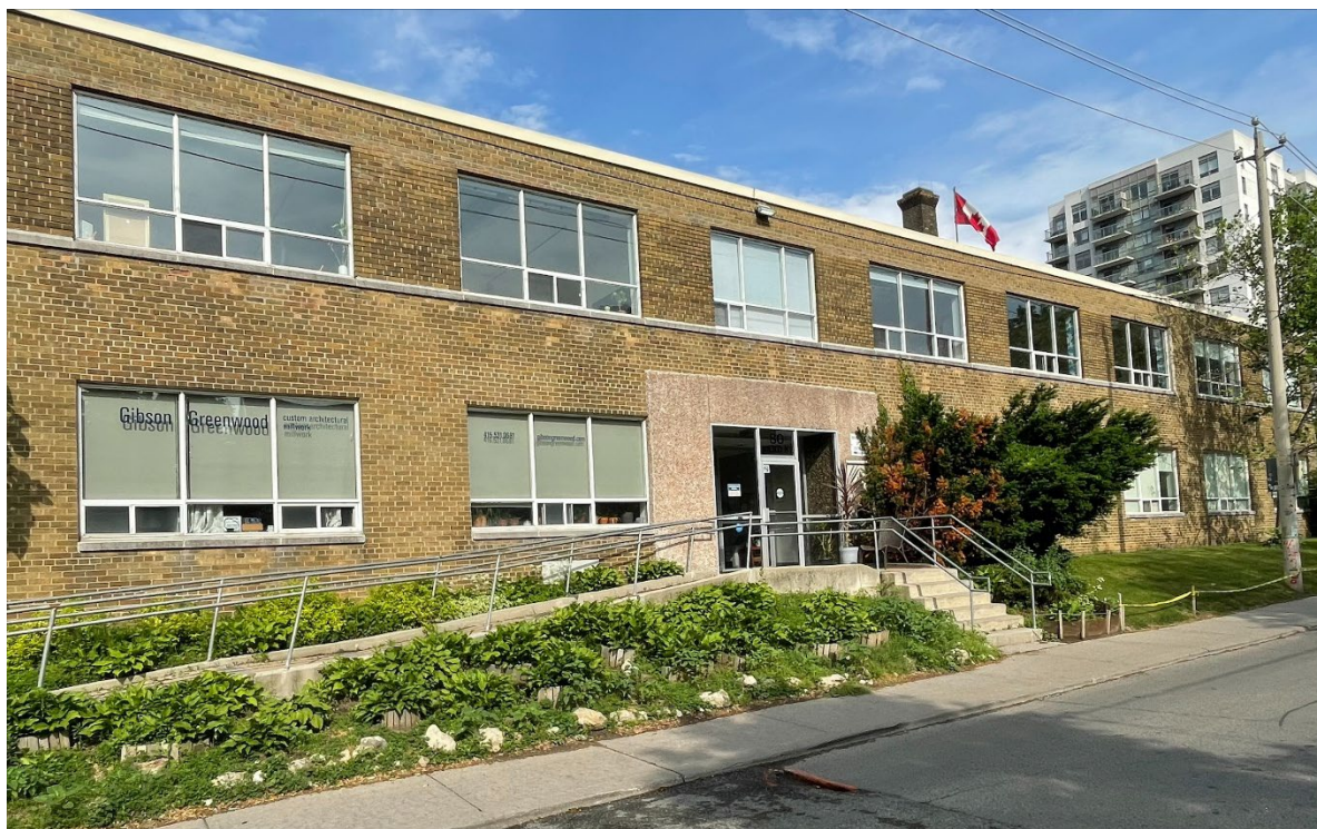
80 Ward Street, principal (east) façade, showing the corporate office portion of the property, 2026 (City of Toronto Heritage Planning, 2026).
