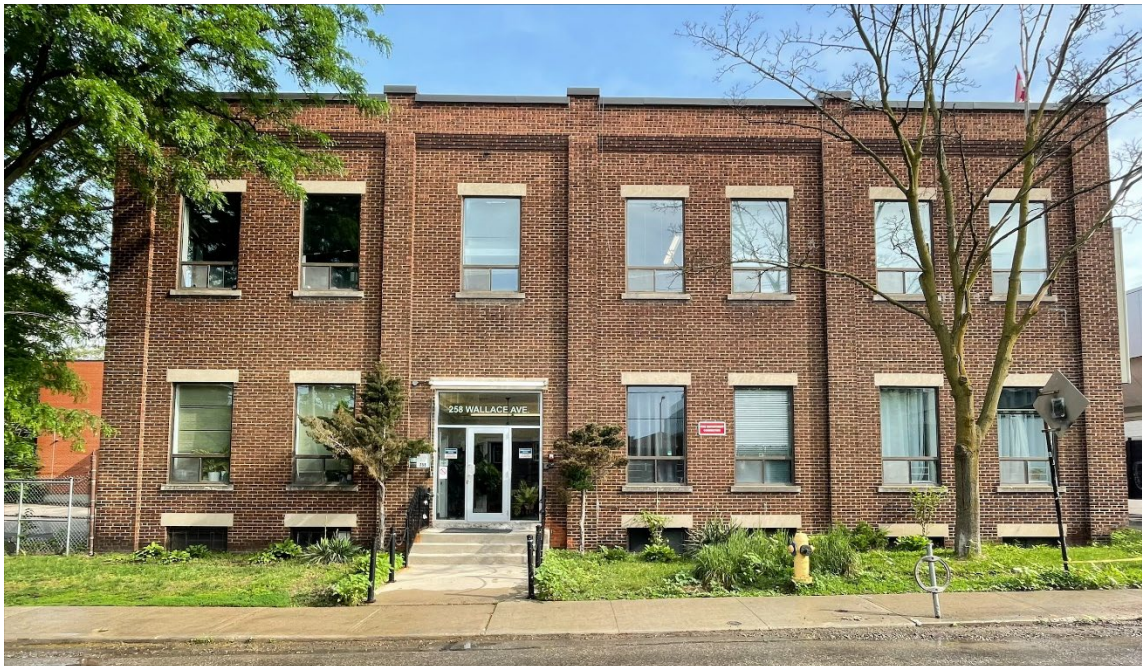
258 Wallace Avenue, principle (south) façade, 2026 (City of Toronto Heritage Planning, 2026)
