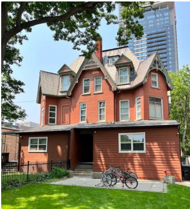
View of 164-166 Isabella Street, showing non-original addition. (GBCA, 2025)
