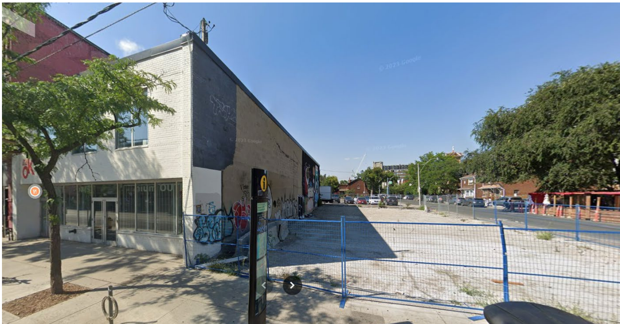
South and East elevations of the subject property at 468 Queen Street West, and the vacant property at 464-466 Queen Street West (Google Streetview 2023).
