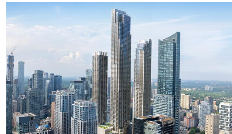
Delivers New Housing While Improving Existing Rental Stock
