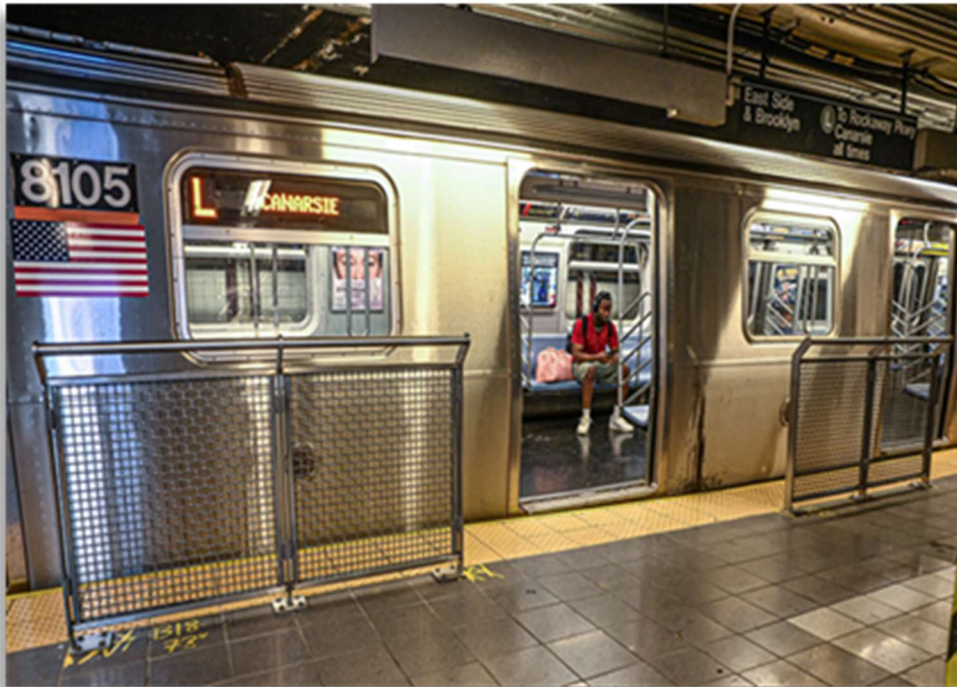
Figure 1: Platform Safety Barriers (Guardrails) installed in New York City
