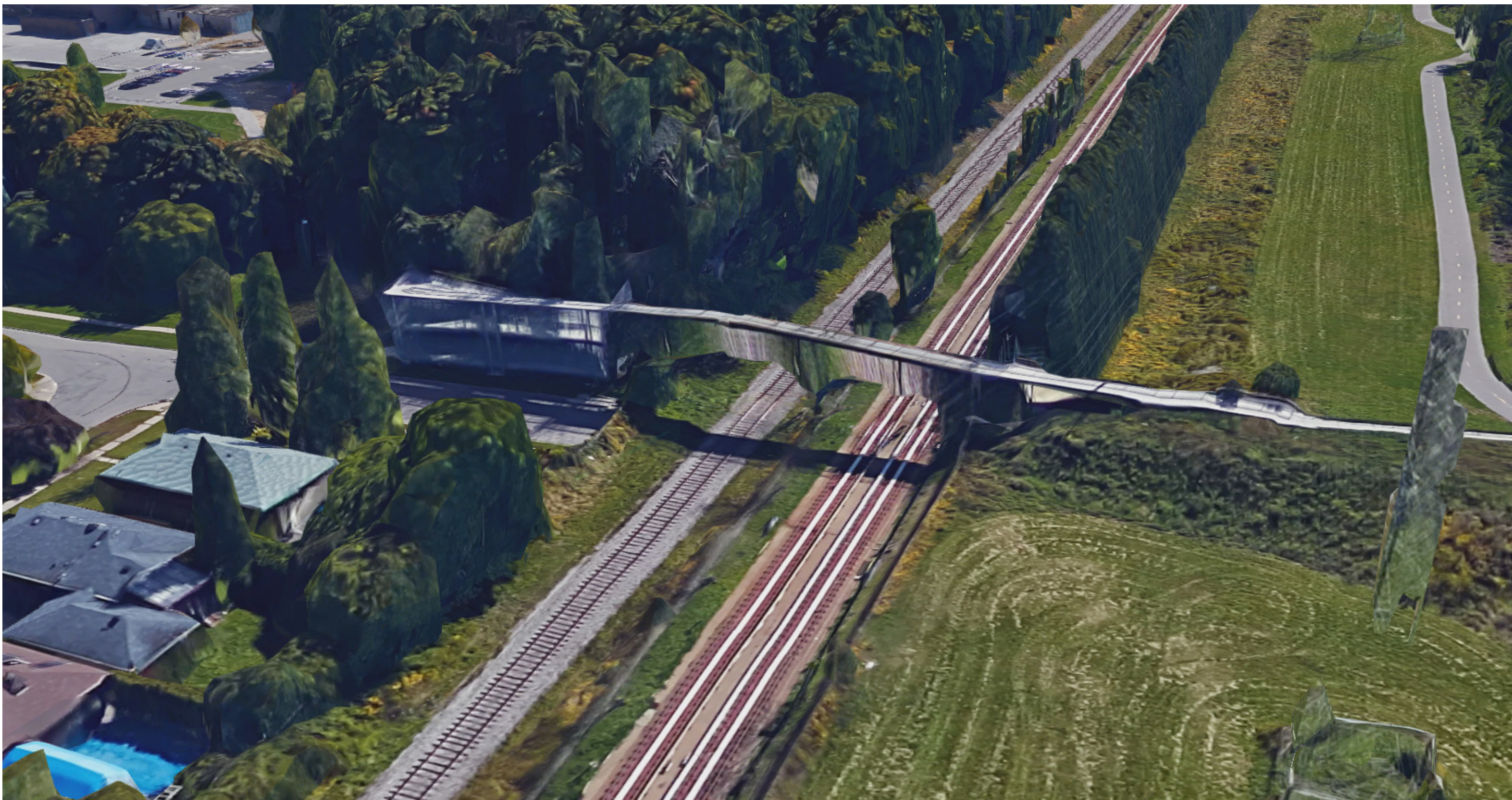
Aerial View Source: Google Maps
