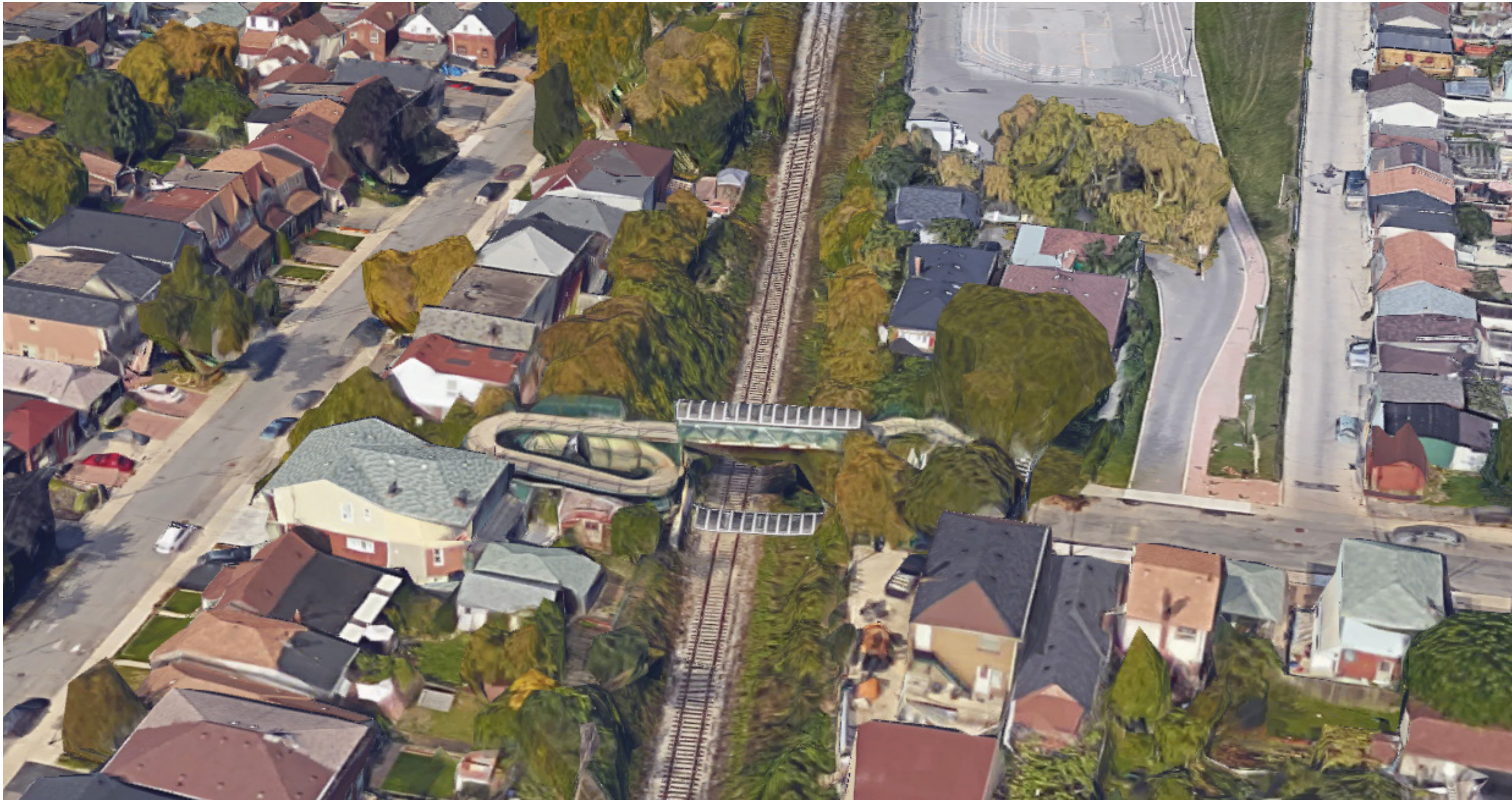
Aerial View Source: Google Maps
