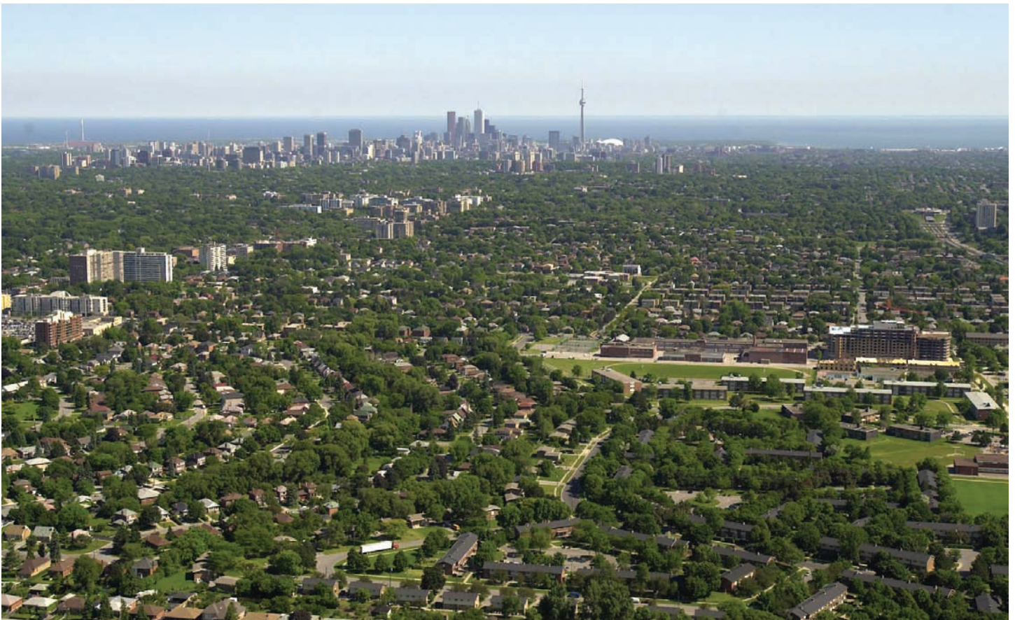
Looking toward Downtown from Allen Road south of Highway 401 - a distance of 10 kilometres to the heart of Downtown.
