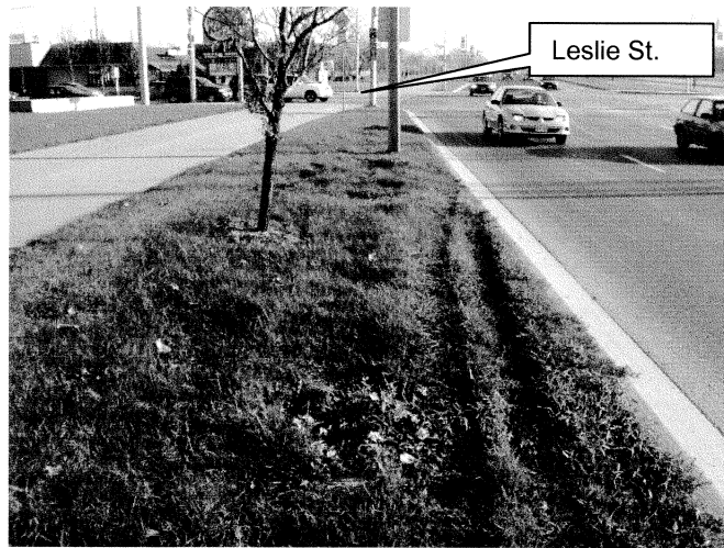
Tire ruts adjacent to north curb of Lakeshore Boulevard.
