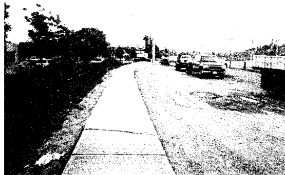
4 – Sidewalk, granular fill and triple mix on far left of photo, Area A.
