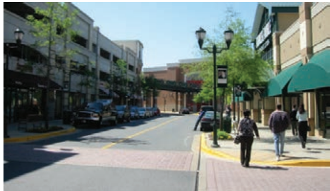
Pedestrian areas should be defined by special paving. Sidewalks should be generous in width to allow for tree grates, pedestrian light standards and other amenities.
