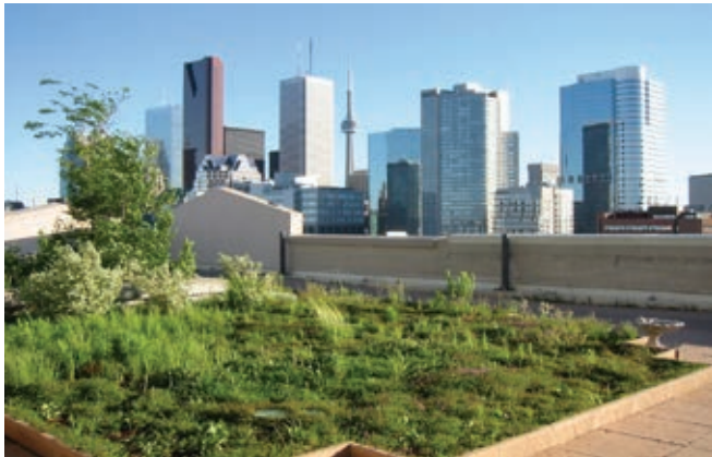
Green roofs provide many benefits, including reducing water run-off and minimizing the urban heat island effect.
