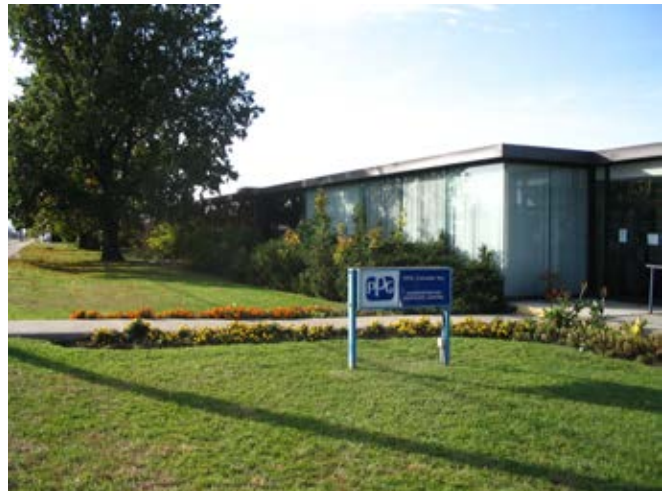
Window's and landscaping enhance the safety and amenity of Caledonia Road.
