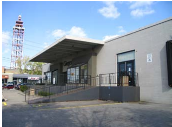
An old loading area canopy provides amenity for a new pedestrian entrance.
