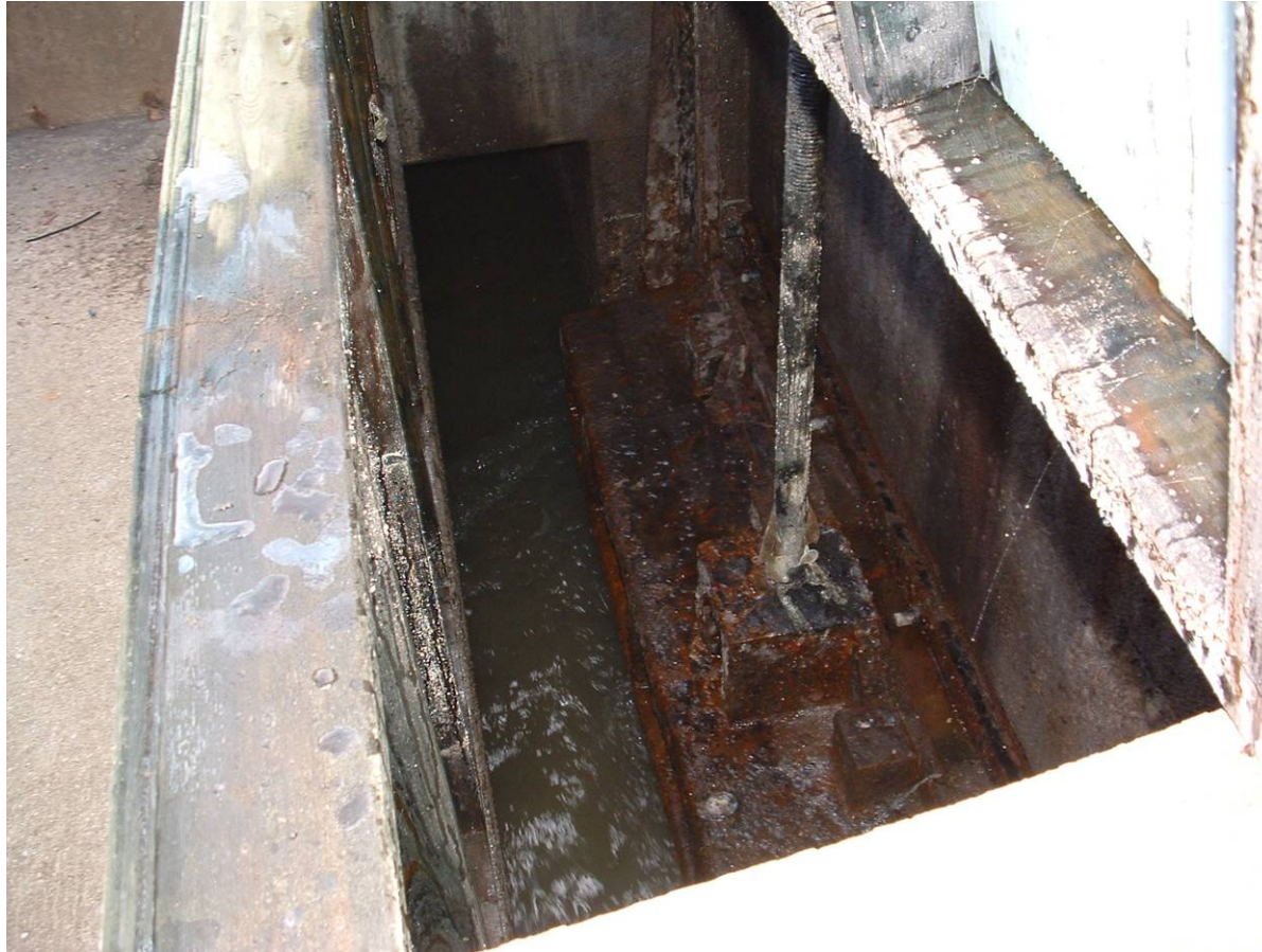
HYDROGEN SULPHIDE CORROSION – INFLUENT BYPASS SLUICE GATE
