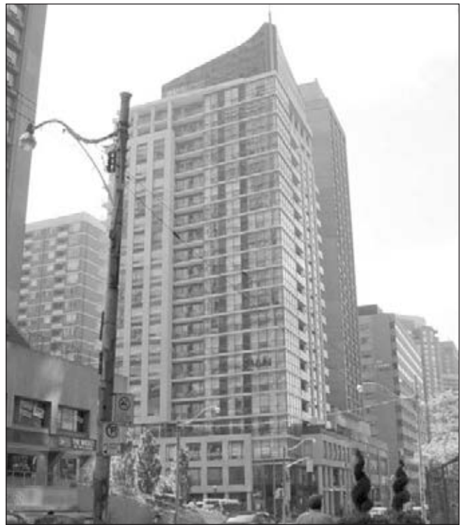
Photo 82 – Roof top mechanical is concealed by architectural features
