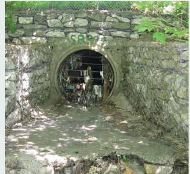
Combined Sewer Overflow Outfall – Taylor Massey Creek photo: Toronto Water
