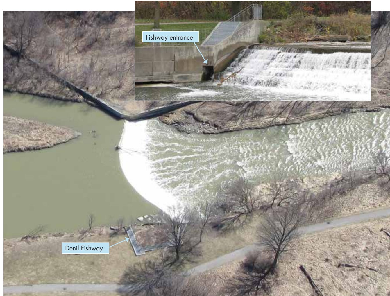
Humber River weir upstream of Eglinton Avenue West. Note the Denil Fishway (a type of fish "ladder") that was constructed to allow both jumping and non-jumping fishes to migrate upstream of the weir (inset shows a side view of the weir and the entrance to the fishway).
