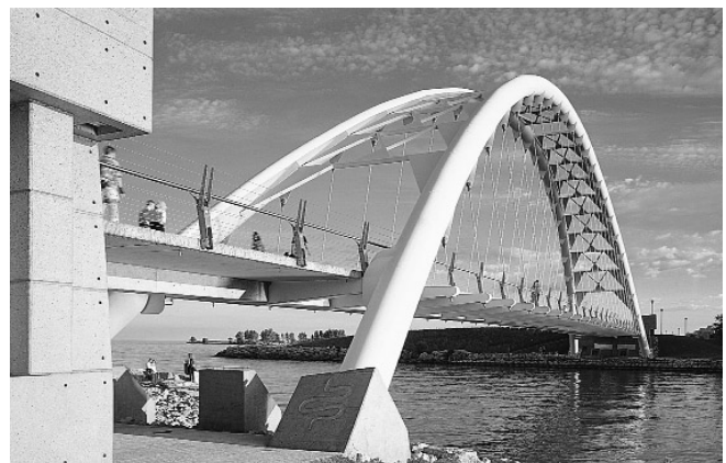
Humber River pedestrian/cycling bridge
