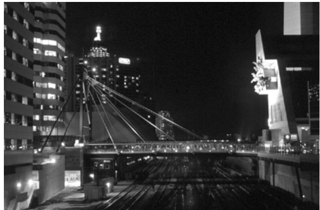
John Street pedestrian bridge: connecting the city to the Railway Lands
