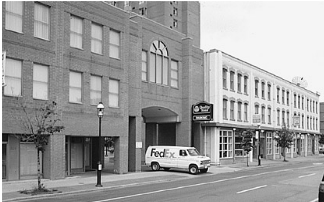
Vehicular service entrance integrated into the street wall
