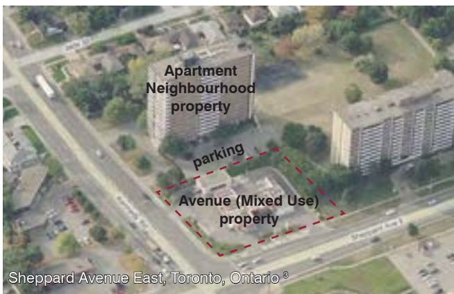
Configuration 1: Where apartment buildings are located parallel to the Avenue's rear property line with a setback that is used as parking or a laneway (example shown at Sheppard Ave. East & Kennedy Rd.). 3
