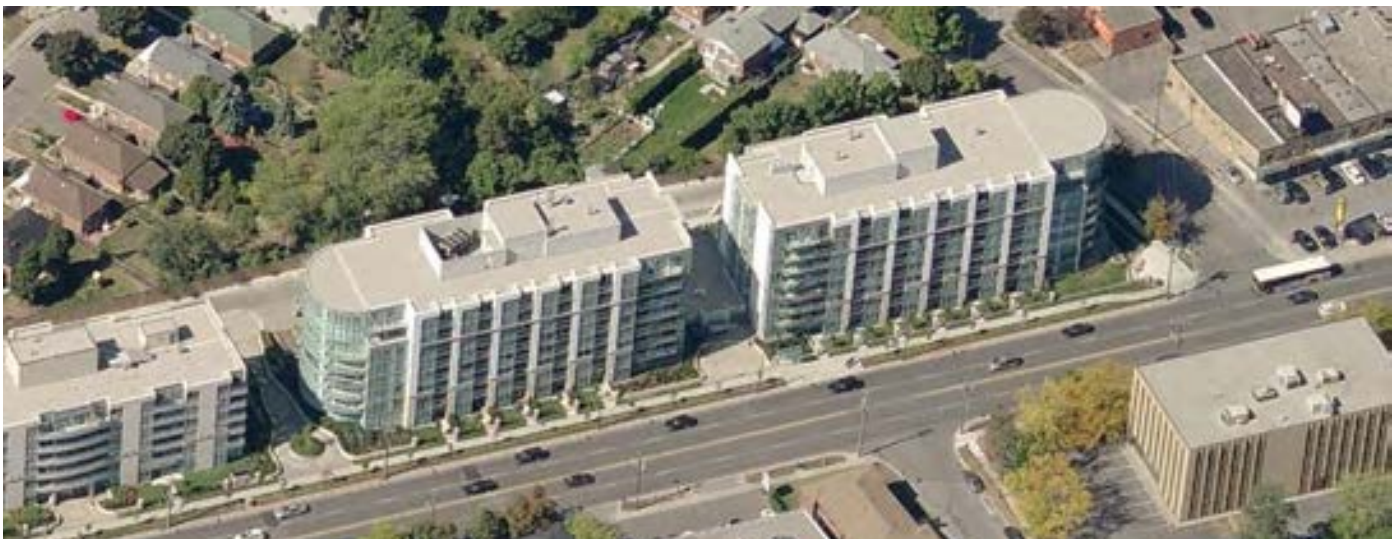
Example of a long building - buildings are broken up to create relief along the Avenue. 9
