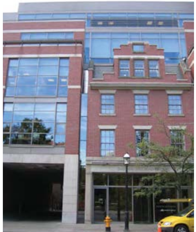
An example of context sensitive façade design and material selection.
