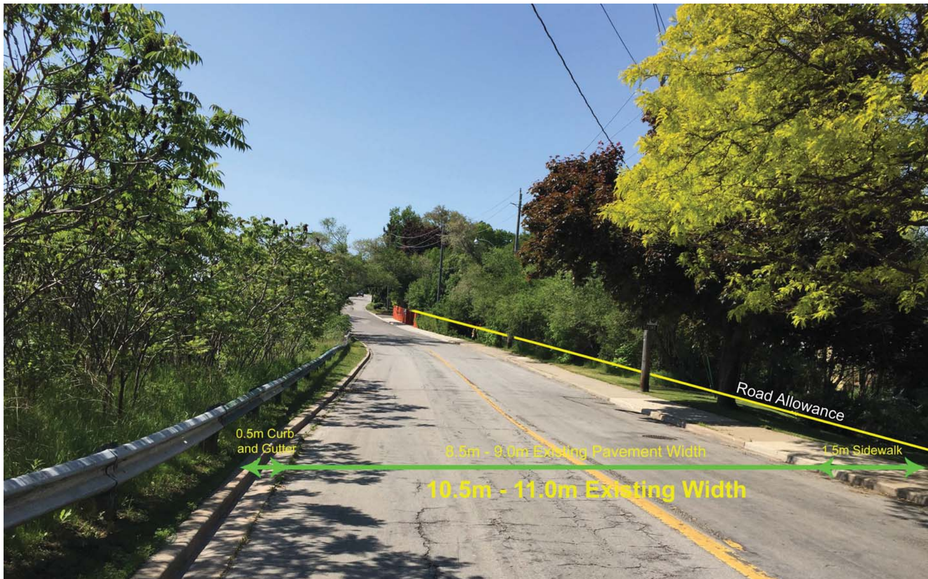
Existing Road Cross Section
