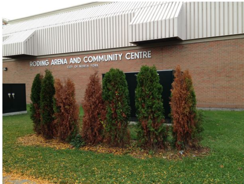
Existing plant landscaping to be maintained by Toronto Hydro reducing visual of Energy Storage Units
