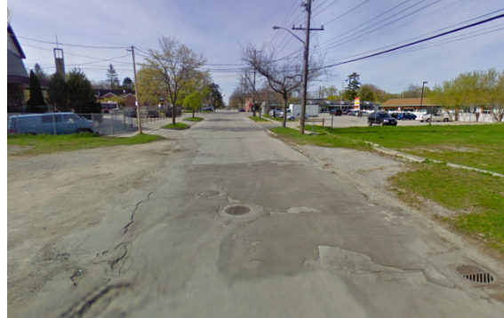
Morrish Road looking north
