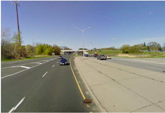
Highway 2A looking east towards the Lawson Bridge
