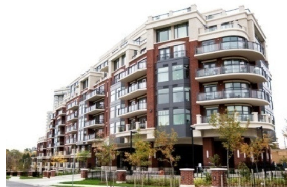
Architectural articulations such as step-backs and change in material are effective measures to reduce a building's scale and minimize its visual impact
