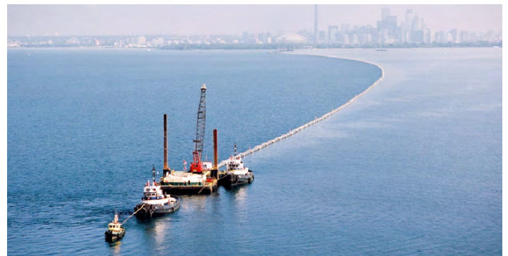
Laying the intake pipe for Downtown's deep lake water cooling system.
