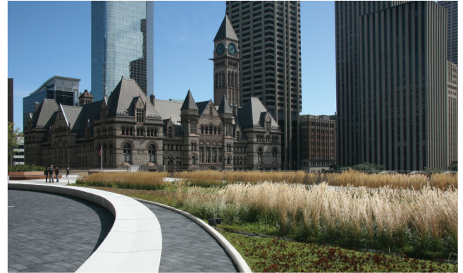
Green Roof at City Hall (Credit: City of Toronto)
