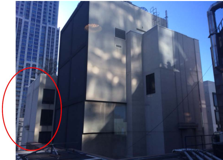
Looking at floors 15-17 of 801 Bay Street taken from balcony of floor 11 of TPS. Looking South
