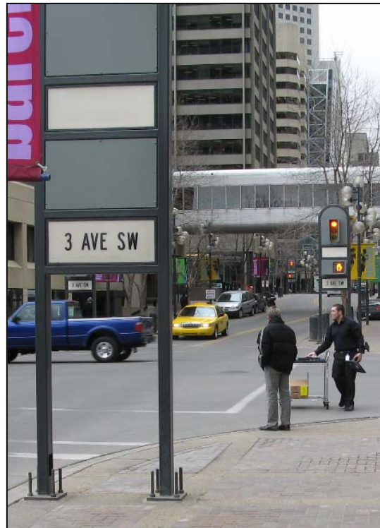
Fig. 9 – Signal Structures on 3 Avenue SW in Calgary
