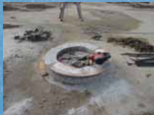
Removed Concrete Riser
