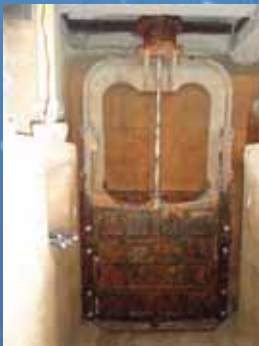
Filter Gate Inside the Filter
