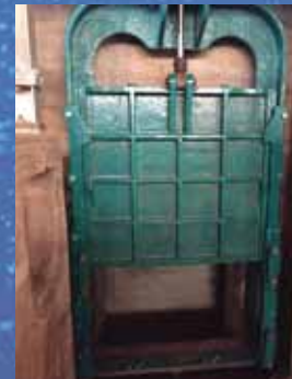
Installed Refurbished Filter Gate
