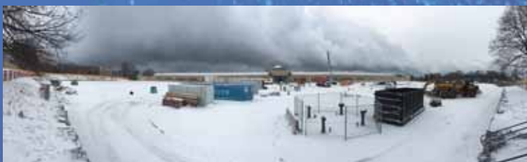
Removal Works on Top of Settling Basins
