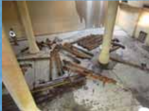
Removal of Existing Cast Iron Wash Down Piping
