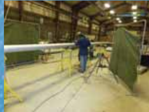
Prefabrication of Stainless Steel Piping Off-Site.
