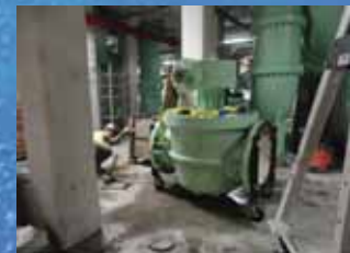
Removed Cone Valve
