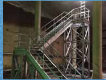
New Access Stair
