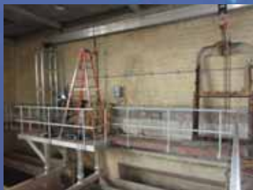
Demounted Gate Frame Lifted Out of the Filter Basin
