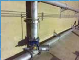
Installed Clean In Place Piping in one of the Basins with Hydraulic Lines and Butterfly Valve
