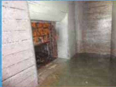
Inlet Gate of Settling Basin, Viewed from the Center Flume Side
