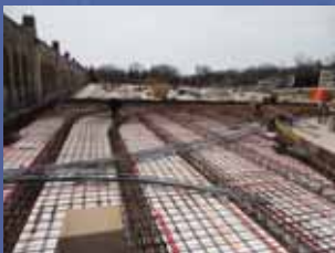
Part of the Rebar for the New Ring Road Including Conduits for Wiring from Filter Building to Field Devices
