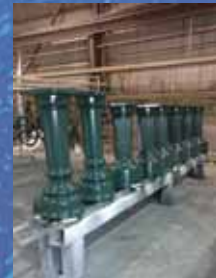
Off-Site Refurbished Pedestals, Ready for Installation
