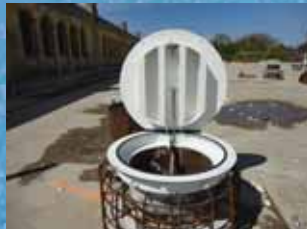
Rebar for Concrete and New Hatch
