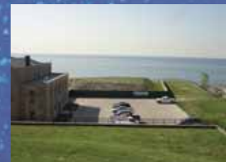
Stockpile Area in Front of Pump Building
