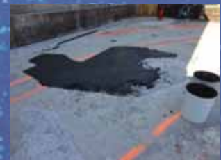
Concrete Repair of Exposed Rebar
