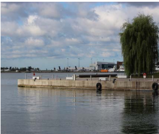
Wharf at HTO Park West
