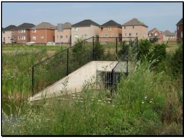
Figure 2-6: Inlet structure of stormwater wet pond (at southwest corner of Staines Road and Seasons Drive)
