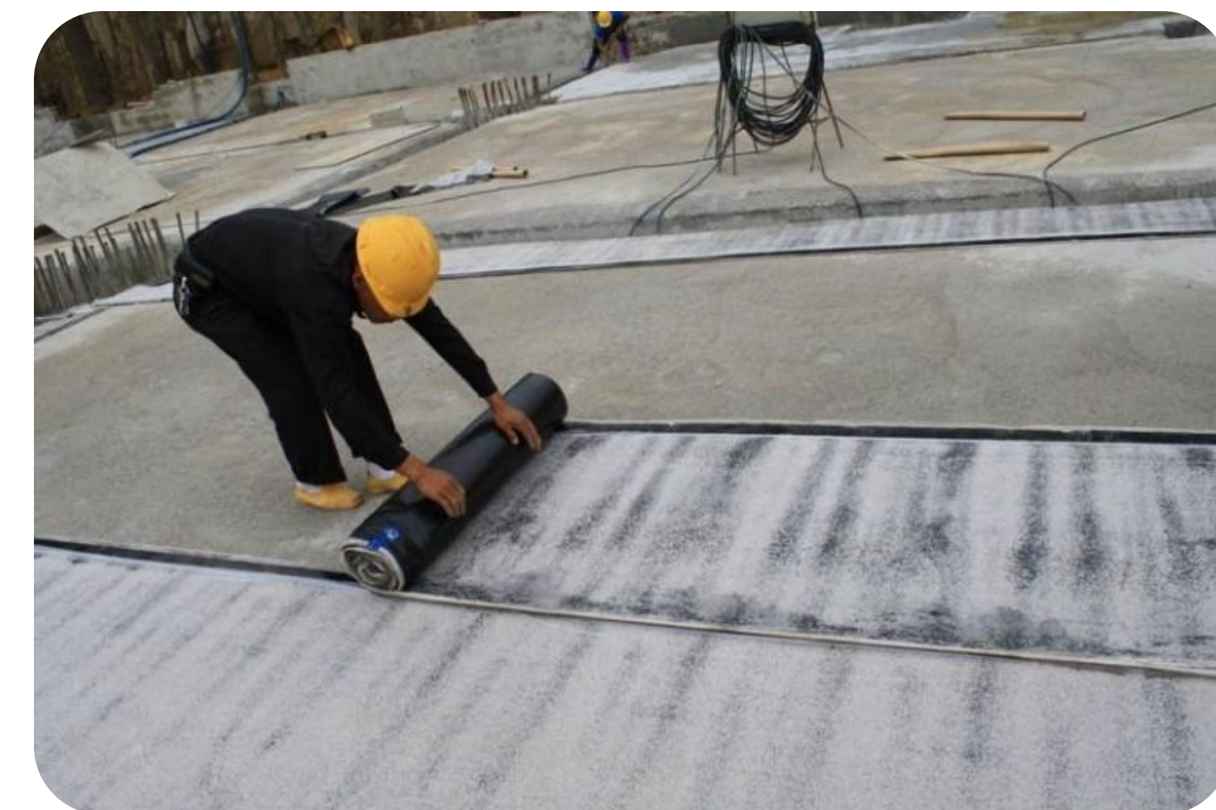
Waterproof Membrane Installation
