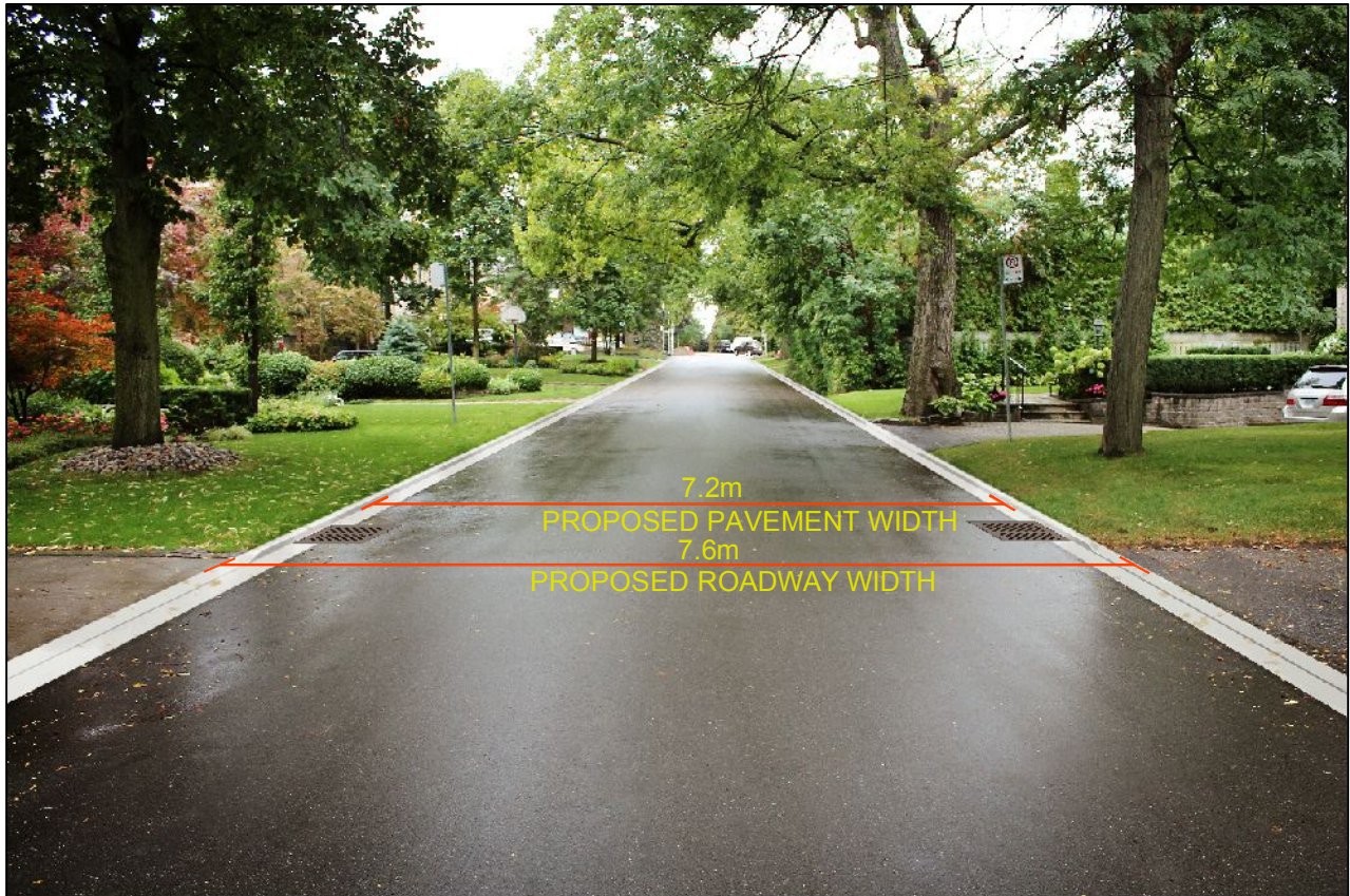
FIGURE BU1 ILLUSTRATION OF EXISTING AND PROPOSED ROAD DIMENSIONS - BUCKINGHAM AVE
