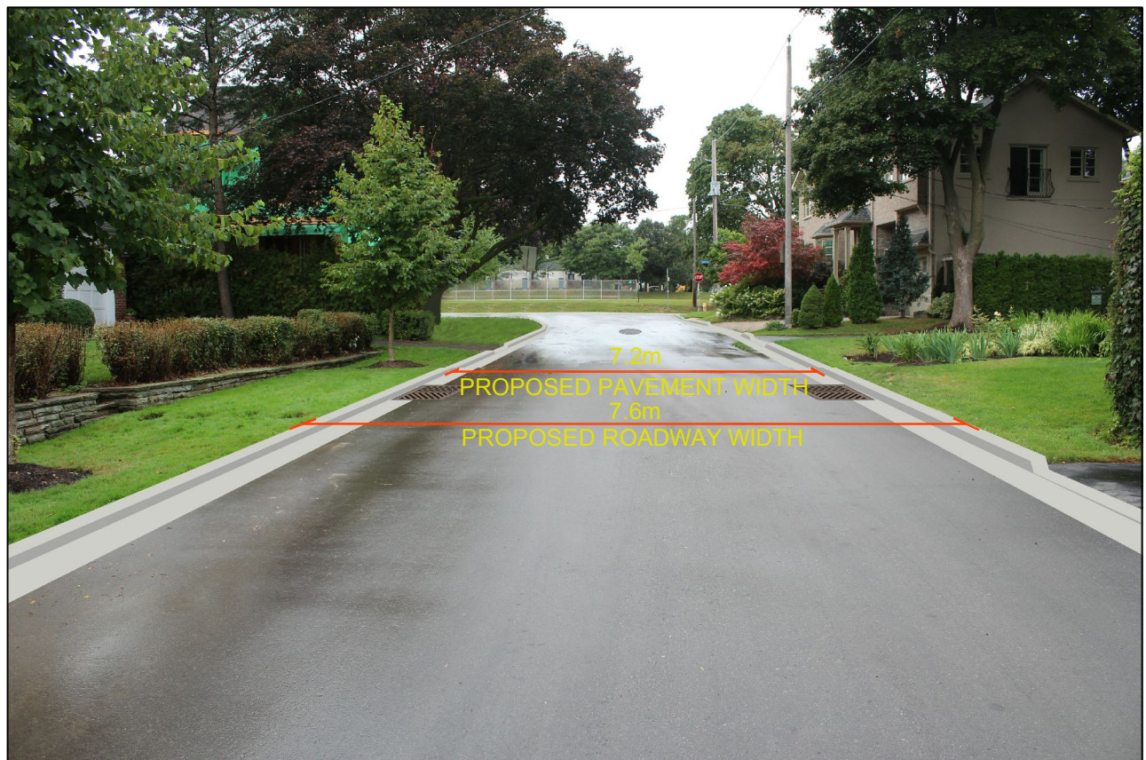
FIGURE BS1 ILLUSTRATION OF EXISTING AND PROPOSED ROAD DIMENSIONS - BRAESIDE CRES
