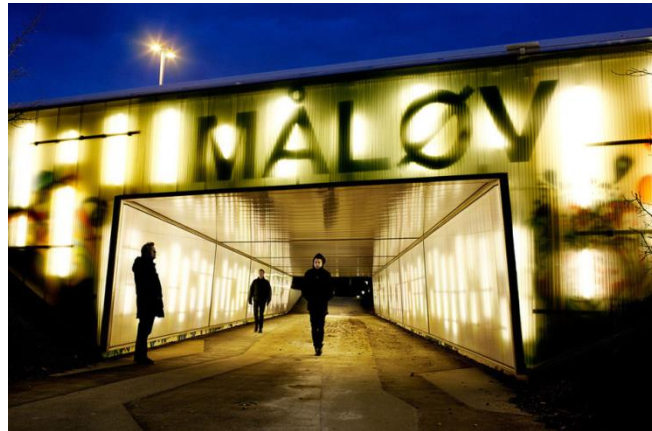
Continuous Lighting in Tunnel
