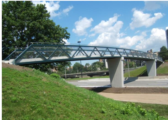
Concrete Steel Truss
