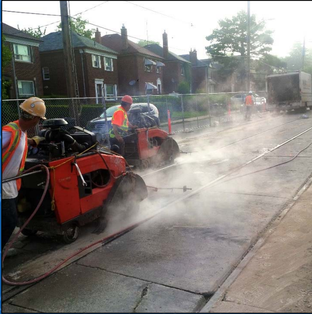
Cutting Concrete
