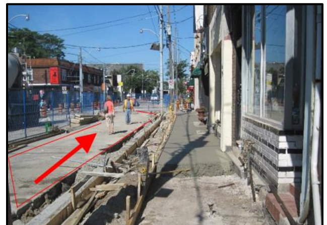
Pedestrian walkway and pedestrian safety fencing at 1.8 metres high, separating the construction zone.
