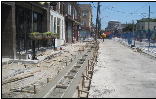
Sidewalk before concrete is poured.
