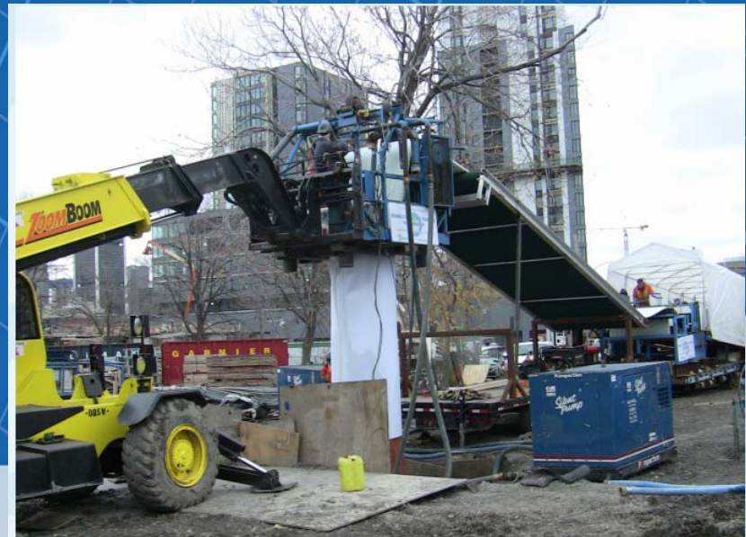
Installation of CIPP liner for a large diameter watermain.
