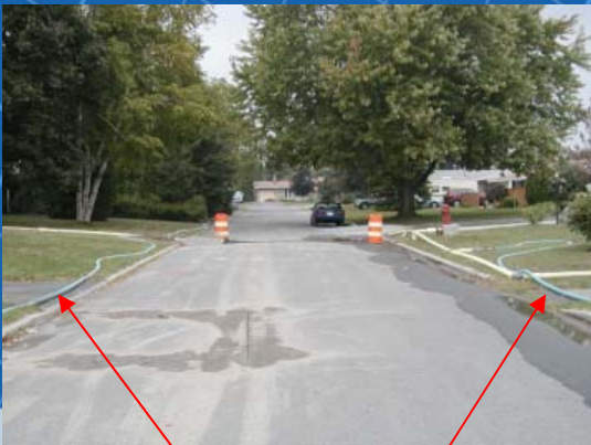
Temporary Watermain Bypass and temporary services laid on street to supply houses with potable water during rehabilitation work.
