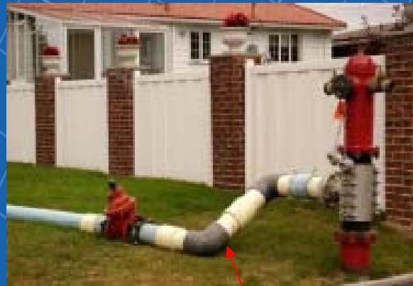
Temporary Watermain Bypass hook-up to existing fire hydrant for water source.
