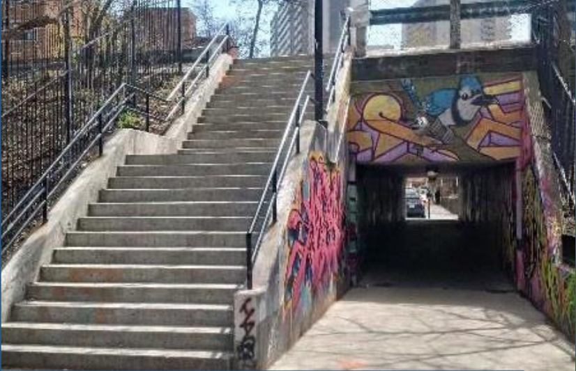
View of tunnel from bridge, looking south
