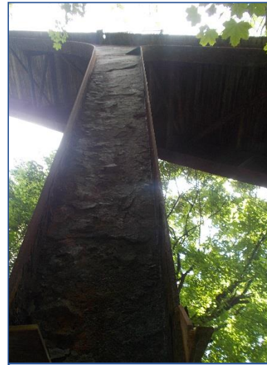
View of corrosion on inclined leg
