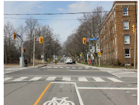
Pavement markings indicate actuated signals for cyclists.
