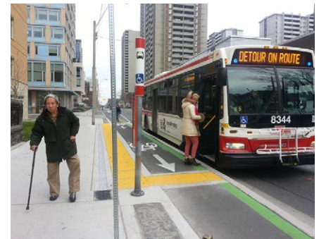
Cycling facility is at sidewalk level for accessible boarding on transit at the intersection.
