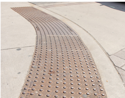
Tactile Walking Surface Indicators are detectable underfoot and used as a warning for people with low or no vision.
