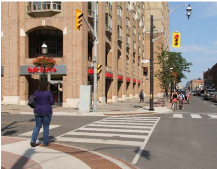
Depressed curbs smooth the transition from sidewalks to roadways.
