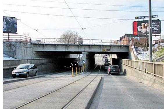
The substructure including the abutments and centre pier use reinforced cast-in-place concrete.
