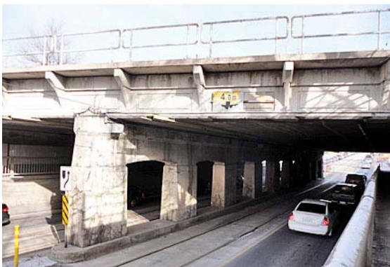
The open spandrel centre pier comprises ten columns connected by a shallow arch.
