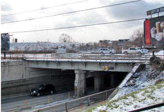
A view southwest to the St. Clair Avenue West Subway depicts the relationship of the railway corridor above and the roadway below.
