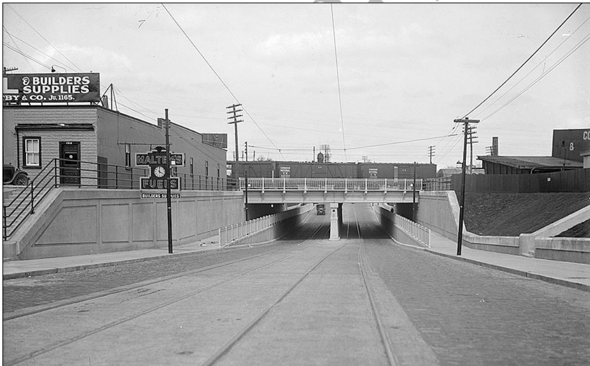
Figure 6. A view east along St. Clair Avenue West depicts the two-span subway structure, retaining walls with stairways and sidewalks [CTA: Series 372, Subseries 63, Item 91, May 19, 1932].
