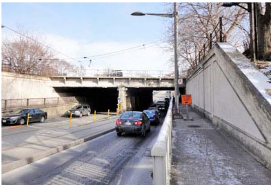
The retaining walls and deck slab structure enclose the roadway as traffic is funnelled into a single lane east of Keele Street.
