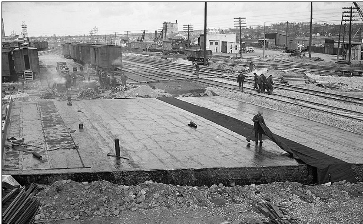
Figure 7. A historical photograph looking northeast across the deck shows the new tracks and ballast at the east side of the bridge and the ongoing waterproofing of the west side of the deck [CTA: Series 372, Subseries 63, Item 76, February 15, 1932].
