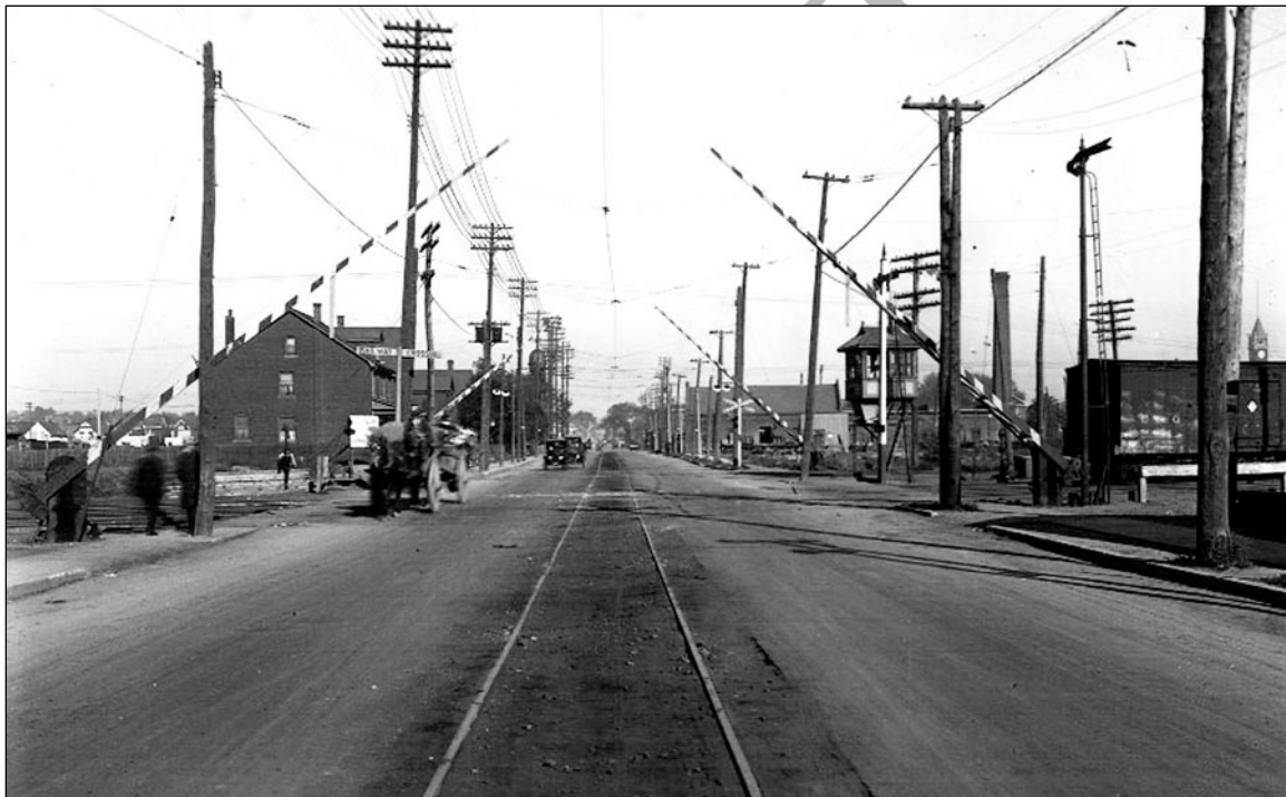
Figure 2. A view east from Keele Street depicts the CN at-grade crossing with gates and watchman's tower on St. Clair Avenue prior to the introduction of the grade separation structure [CTA, Fonds 1231, Item 2042, October 8, 1923].
