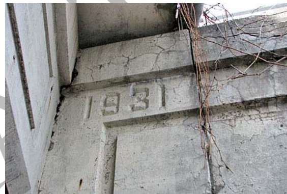
The construction date of 1931 cast at the east end of the north abutment relates to the completion of the substructure work.
