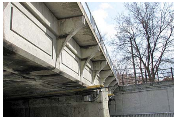
The brackets support the walkway located on the outside of the deck. Rectangular panel detailing highlights the visible side of the deck slab.
