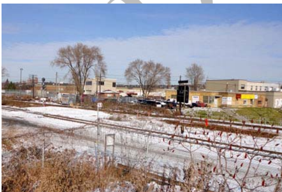
The railing at the edge of the deck is the only distinguishing feature that locates the bridge along the rail corridor.
