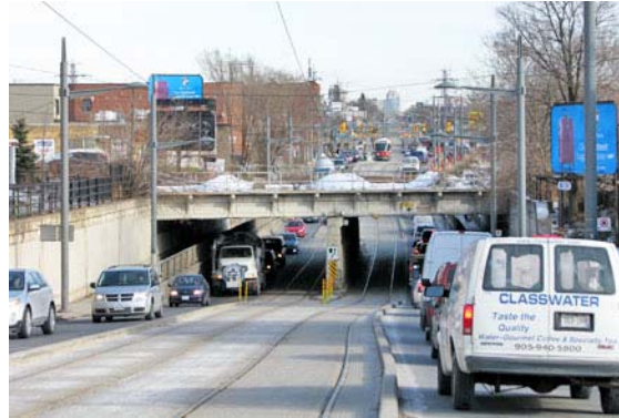
The dedicated streetcar right-of-way runs along the centre lanes of the four-lane St. Clair Avenue West.
