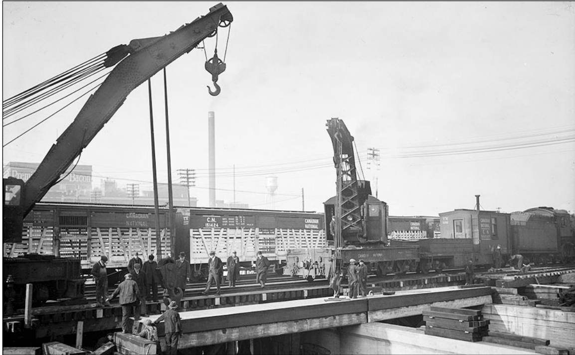
Figure 4. A photograph of the St. Clair Avenue West Subway shows the wrecking cranes in position to lift the concrete deck slabs into position on the abutments and centre pier [CTA: Fonds 200, Series 372, Subseries 63, Item 67, January 8, 1932].
