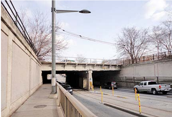
A view of the west side of the St. Clair Avenue West Subway depicts the general arrangement of the two-span, precast concrete deck slab structure.
