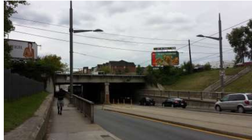
IMAGE 6: Looking slightly southwest on St. Clair Ave W at disturbance associated with paved areas (road, sidewalk) and railway underpass within Option 1
