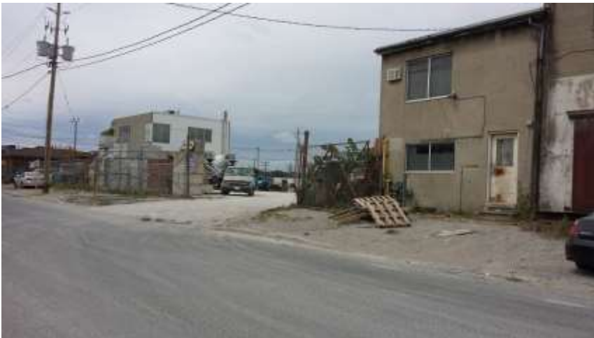
IMAGE 35: Looking northwest on Townsley Street at disturbances associated with grading, paved road and parking lot, utilities and existing buildings within Option 4.
