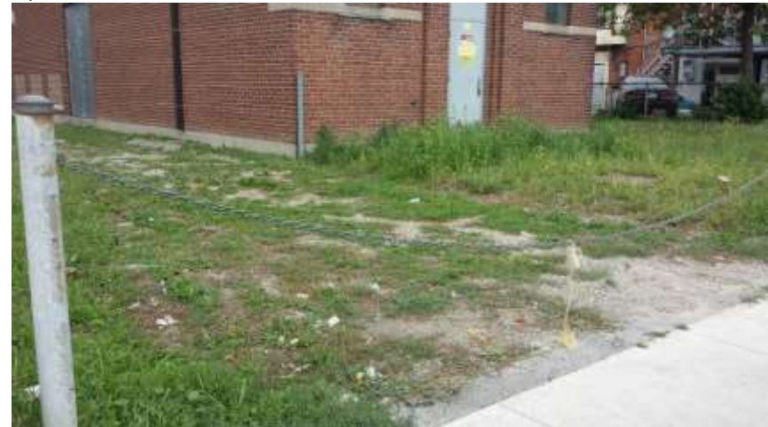
IMAGE 8: Looking northeast on St. Clair Ave W at disturbances associated with TTC utility building, grading, and paved sidewalk within Option 1.
