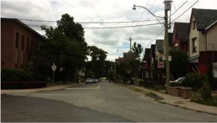
IMAGE 25: Looking slightly southeast at Mullock Avenue and disturbances associated with paved road and sidewalks, existing buildings and utilities within Option 3.
