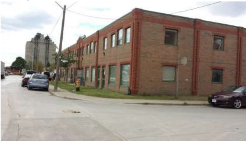
IMAGE 27: Looking south on Cawthra Avenue at disturbances associated with existing buildings, paved areas (road, sidewalk) and utilities within Option 3
