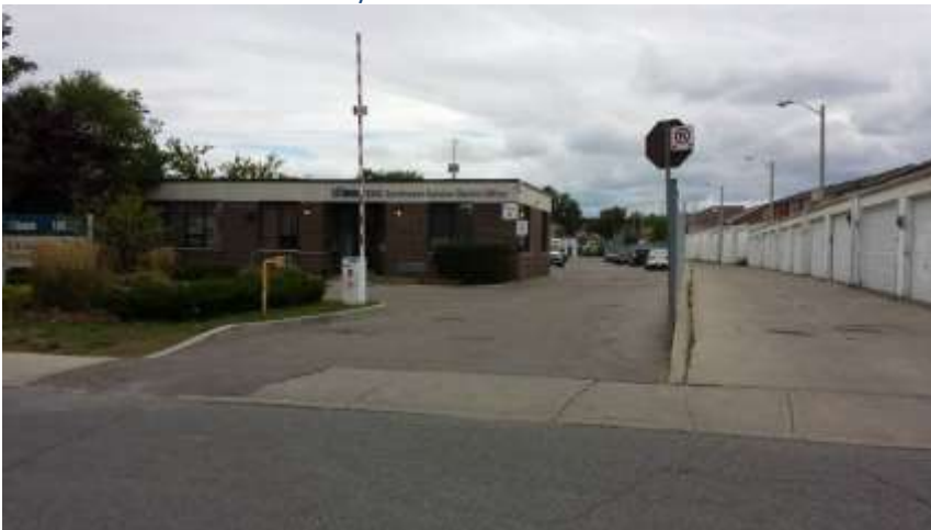
IMAGE 15: Looking northwest on Turnberry Avenue at disturbances associated with EMS building, garage structures, paved road, parking lot and sidewalk within Option 2
