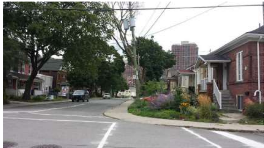
IMAGE 28: Looking slightly southeast at Mullock Avenue and disturbances associated with paved road and sidewalks, existing buildings and utilities within Option 3.
