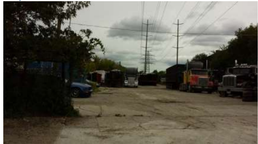
IMAGE 36: Looking slightly northeast on Union Street at disturbances associated with paved parking lot and utilities within Option 4.
