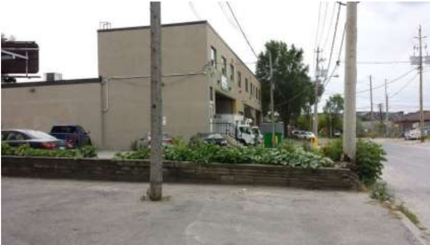
IMAGE 9: Looking slightly southwest on Townsley Street at disturbances associated with existing buildings, paved areas (parking lot, driveways, road) and utilities within Option 1
