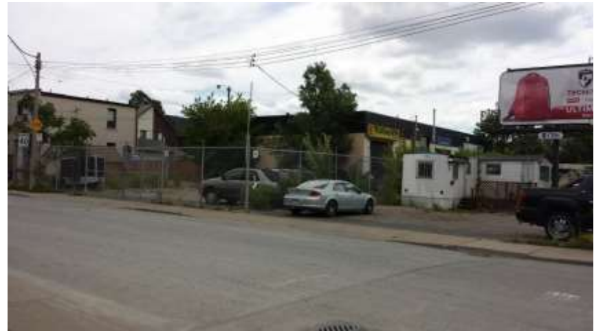
IMAGE 24: Looking southeast on Lloyd Avenue at at disturbances associated with existing buildings, paved areas (parking lot, road, sidewalk) and utilities within Option 3
