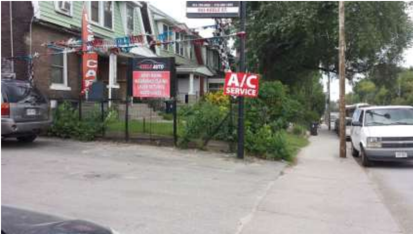
IMAGE 29: Looking slightly southeast on Keele Street at disturbances associated with existing buildings, paved areas (road, sidewalk, parking lot) and utilities within Option 3
