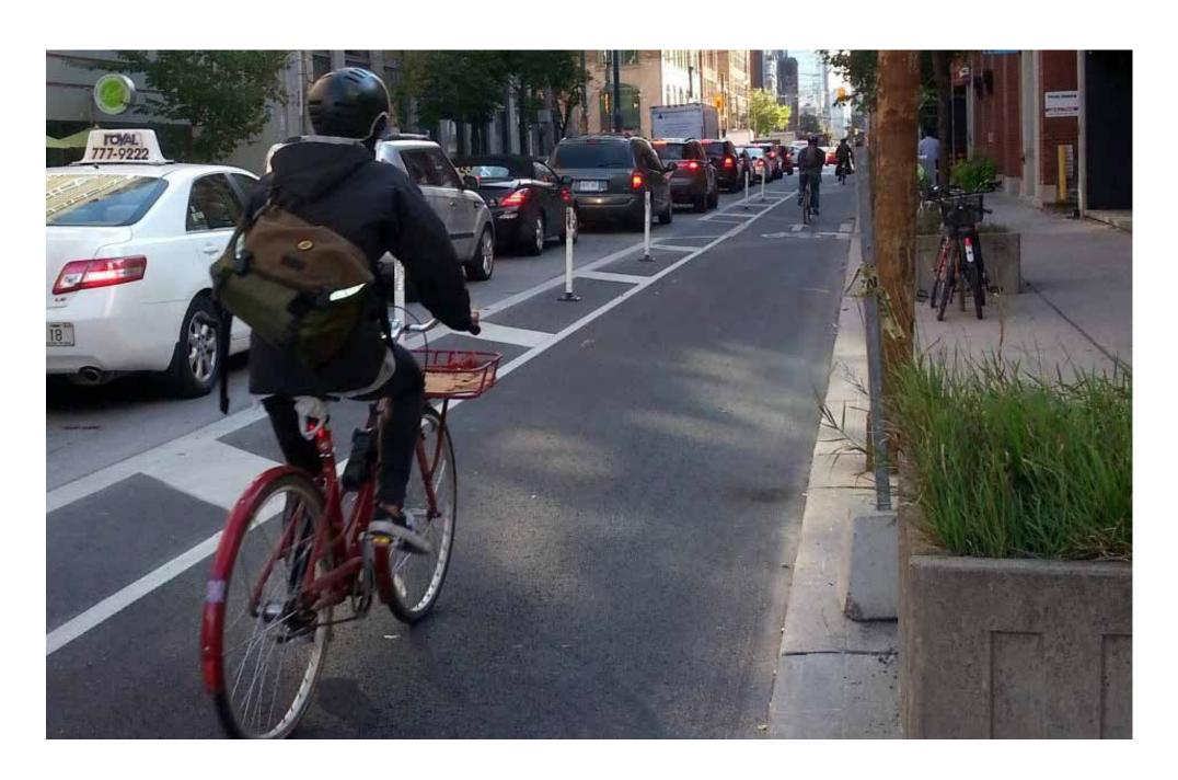
**Cycle Track:** Features separation elements, such as parked cars and flexiposts, between the bike lane and the traffic lane, as well as between the bike lane and parked cars ("door zone").
