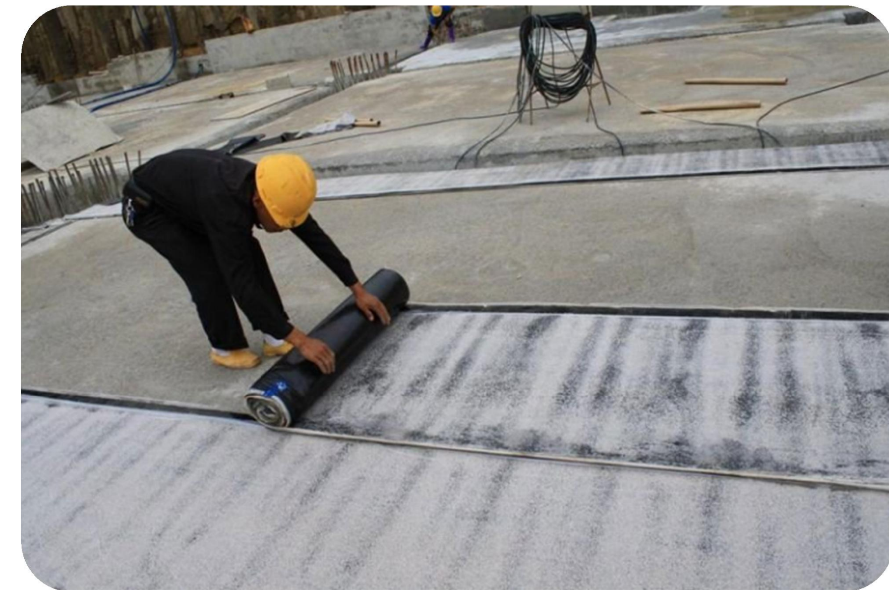
Waterproof Membrane Installation
