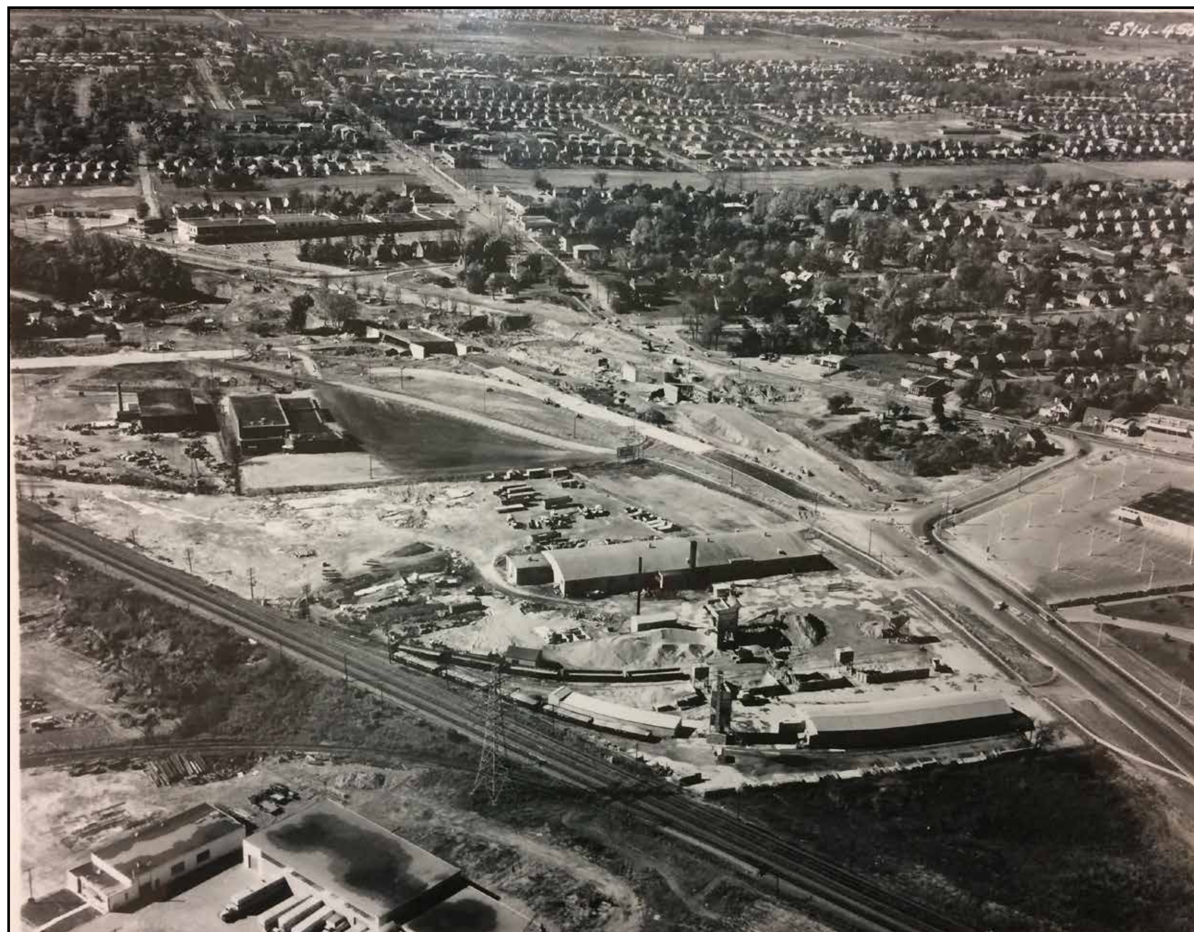
Looking east, along CPR at Kipling Station, 1982
