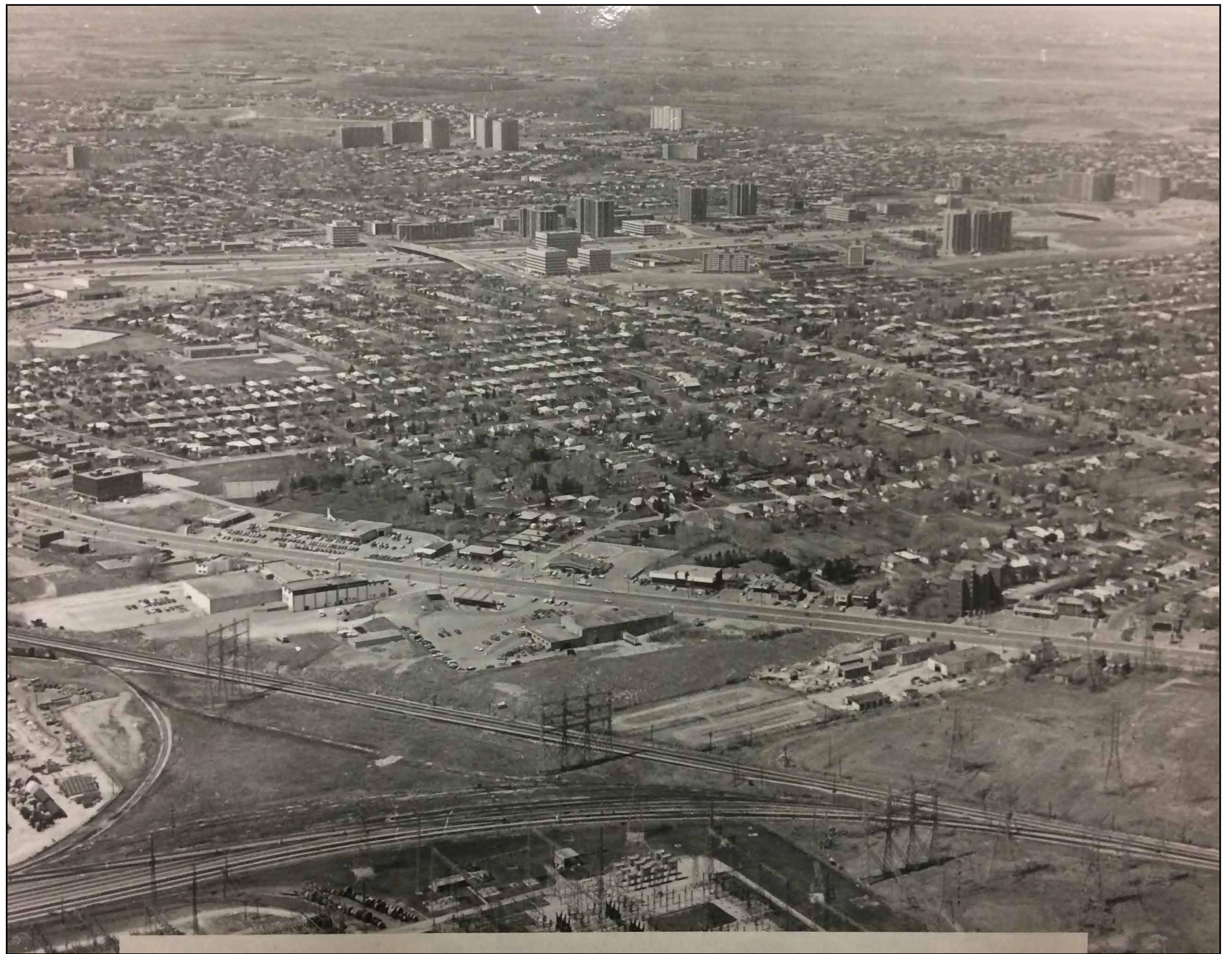
Site of Kipling Subway Station, 1978
