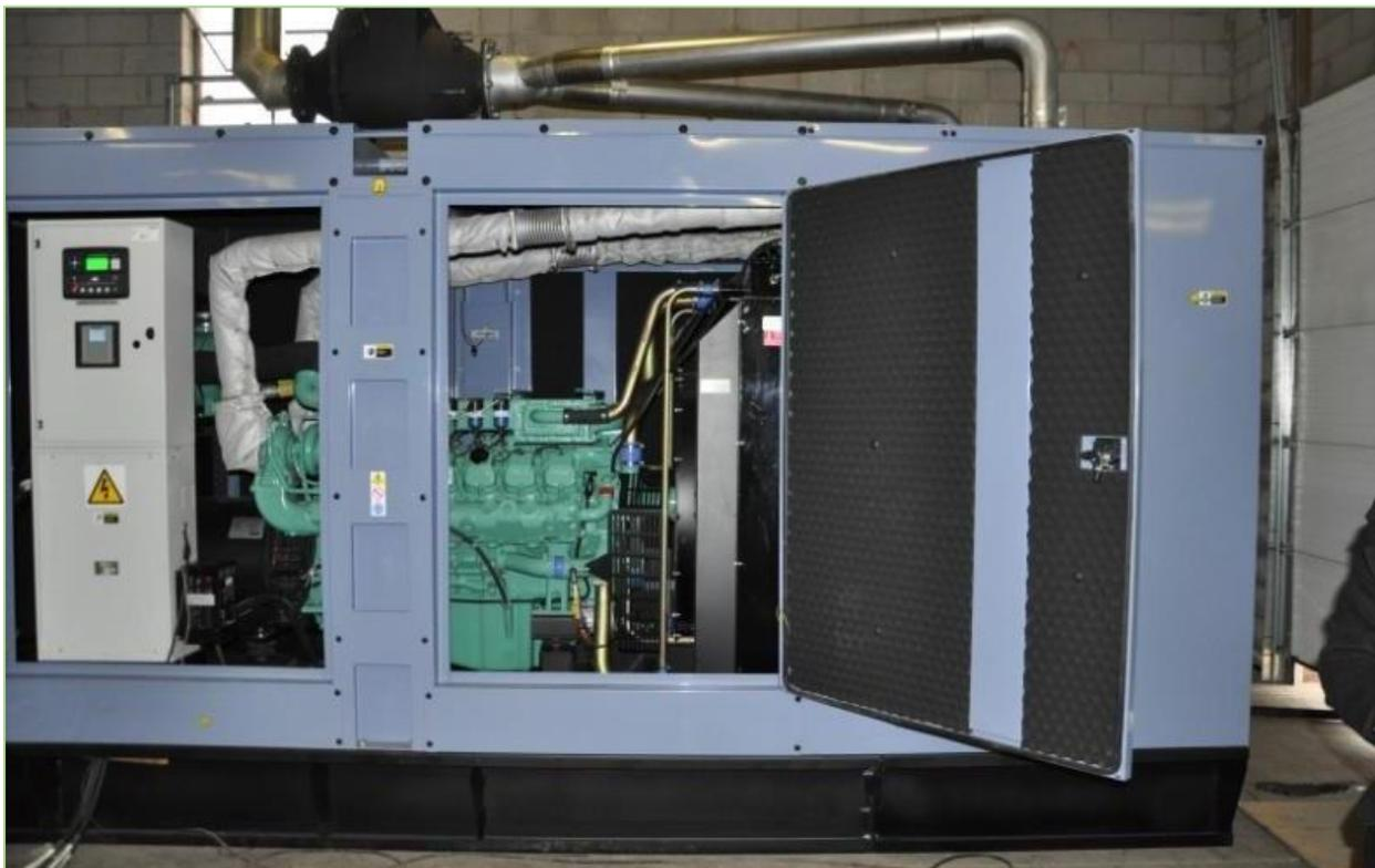
**Packaged, 400 kW natural gas-fired generator.**
