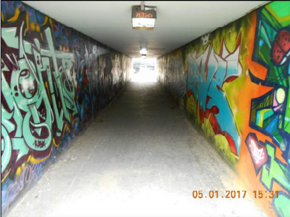
Photo 5: Typical Tunnel Barrel
