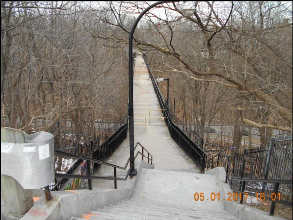
Photo 20: Pedestrian Bridge North of Tunnel
