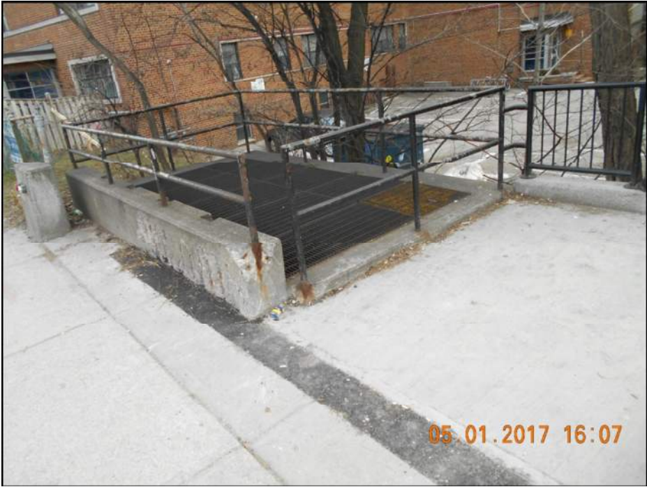
Photo 11: TTC Vent Shaft to Southeast of Tunnel
