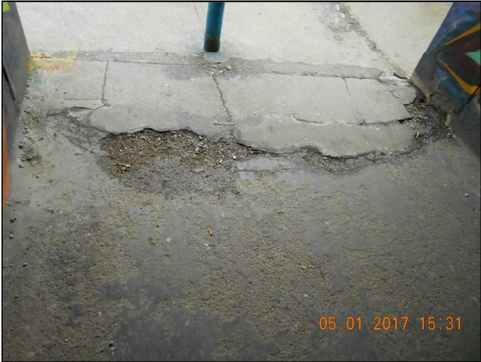
Photo 23: South Entrance Floor Slab
