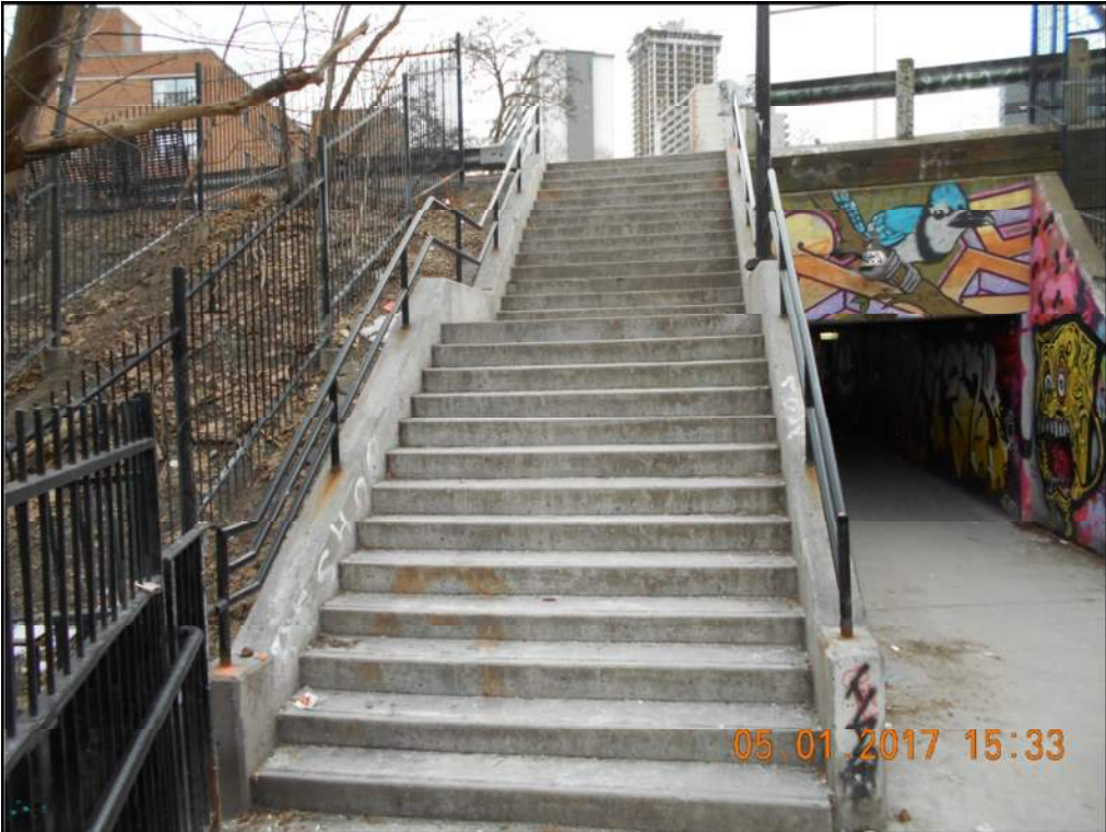
Photo 4: Stairs from North Entrance to Bloor Street
