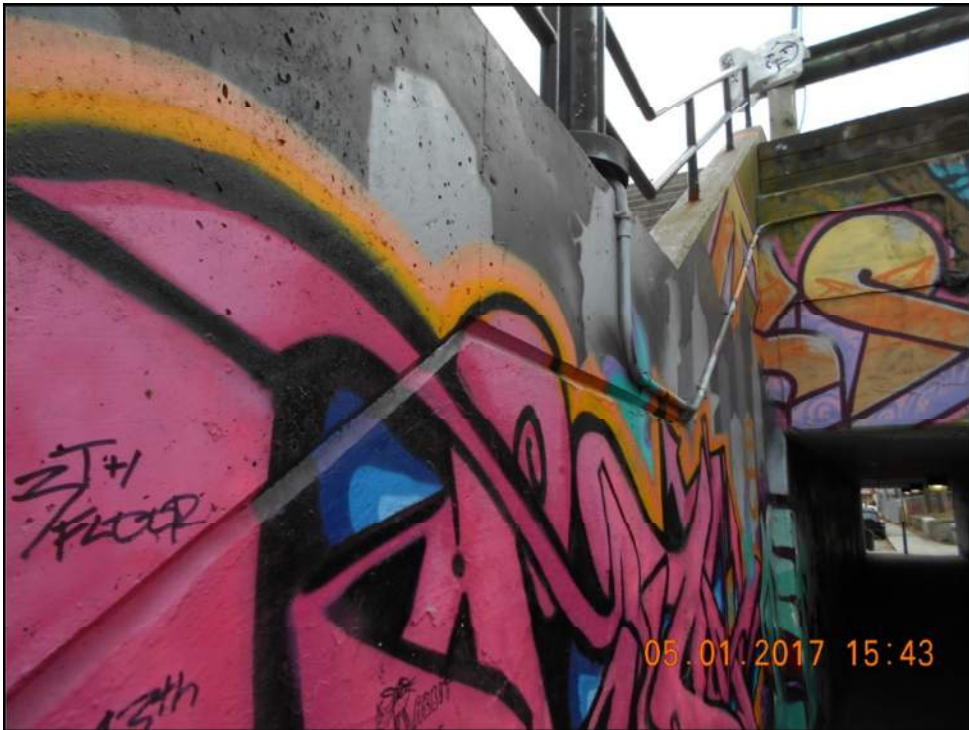
Photo 21: North Stairs Wall (Newer Concrete Curb)
