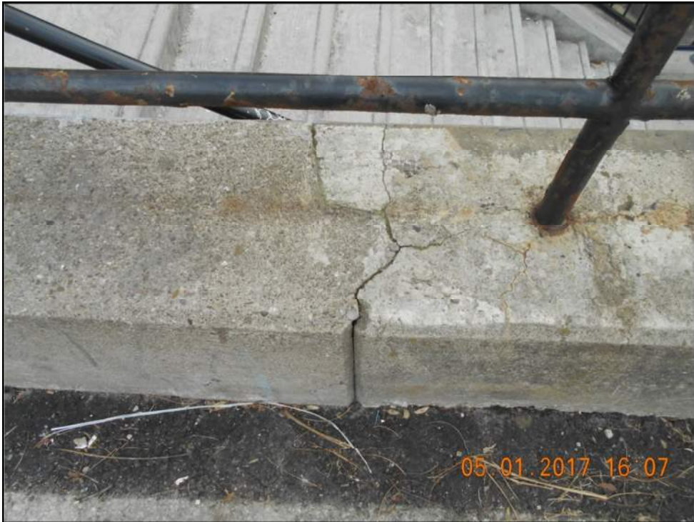
Photo 24: Construction Joint in South Retaining Wall and Typical Railing Condition
