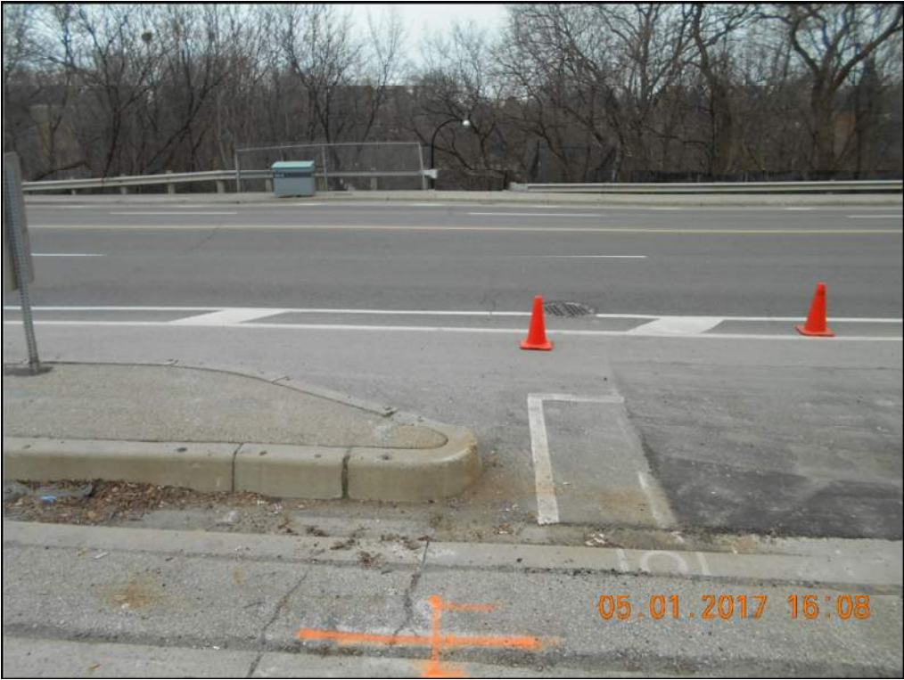
Photo 8: Asphalt Wearing Surface above Tunnel (looking north)
