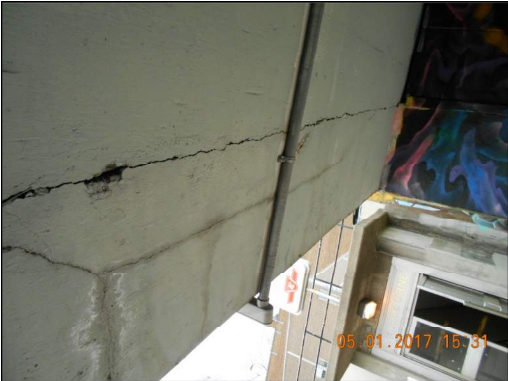
Photo 16: South Entrance Soffit
