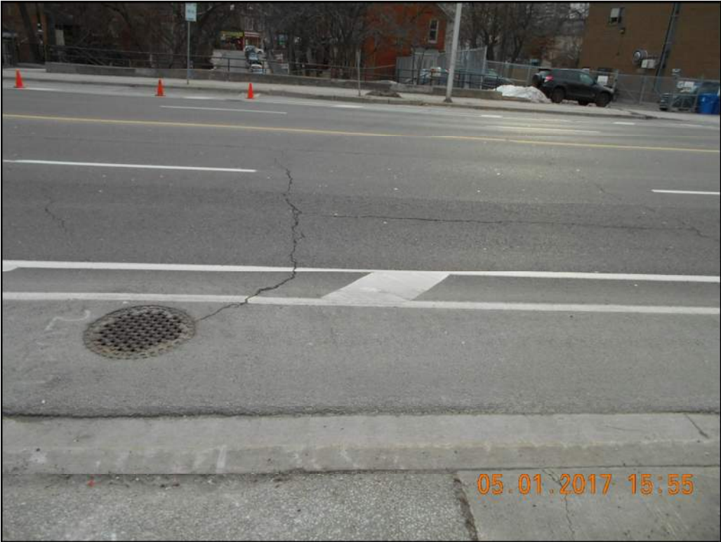
Photo 7: Asphalt Wearing Surface above Tunnel (looking south)
