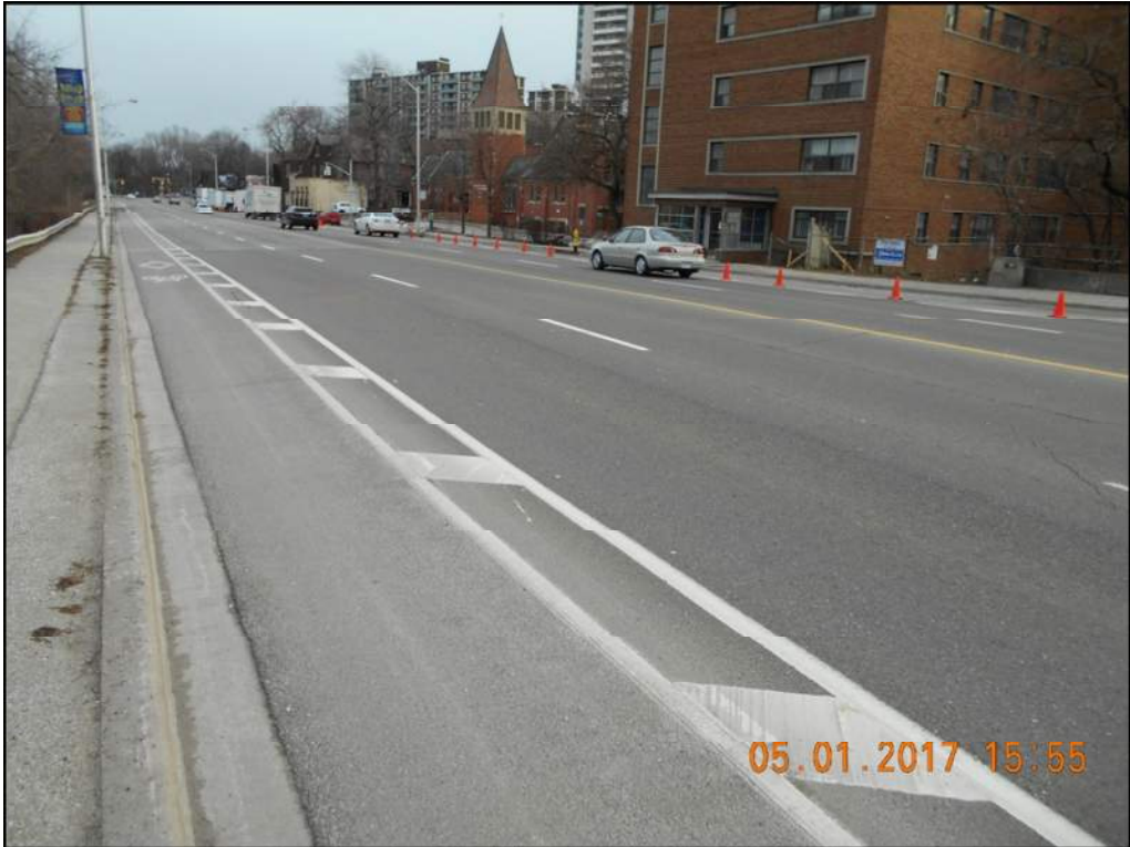
Photo 14: Looking East above the Tunnel (on Bloor Street)
