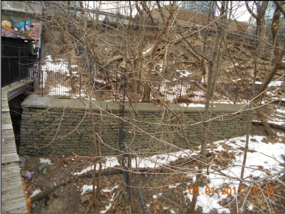
Photo 10: Northwest Embankment and Retaining Wall
