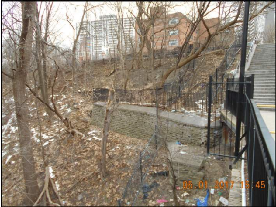
Photo 9: Northeast Embankment and Retaining Wall
