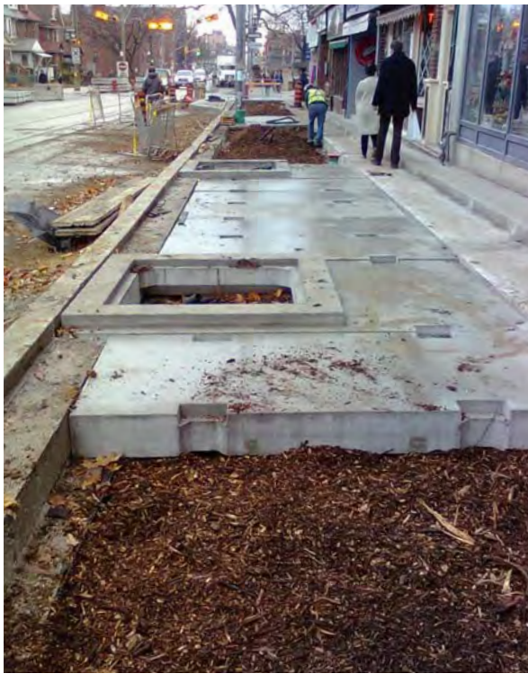
Figure 21 - Roncesvalles Boulevard during sidewalk reconstruction and after
