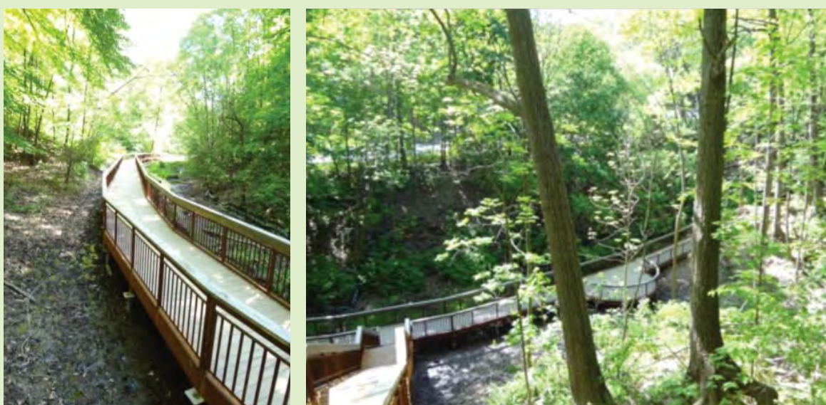
Figure 27 - Glen Stewart Ravine boardwalk and staircase designed to limit user impacts on seepage area and sandy slopes.
