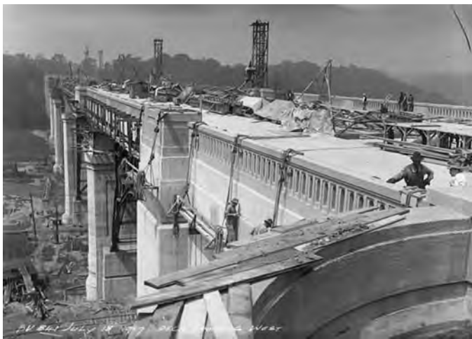
Figure 2 - Construction of the Bloor Viaduct, 1917.
