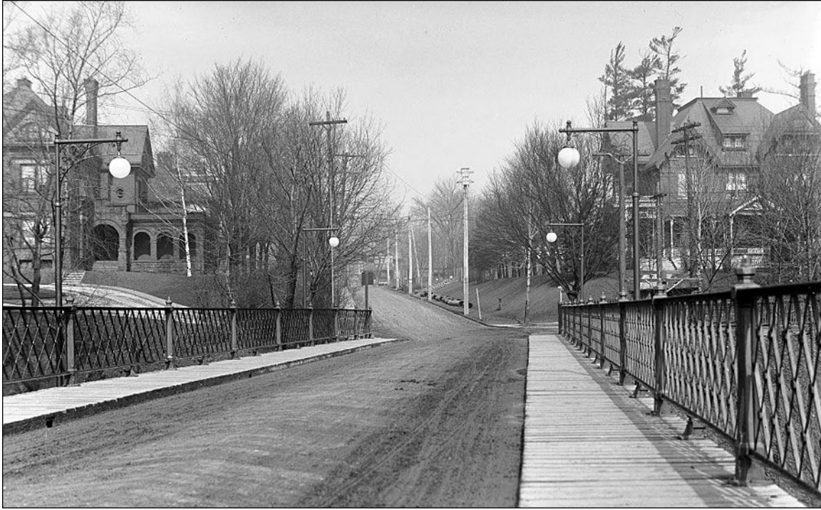
A view north across the Glen Road Bridge illustrates the wood sidewalks, the lattice railings and the pendant style street lighting [CTA, Fonds 200, Series 372, Subseries 10, Item 79, March 14, 1913].
