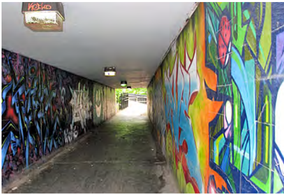
The concrete box structure of the tunnel has a cement floor, concrete ceiling with four light and glazed wall tiles covered with graffiti.
