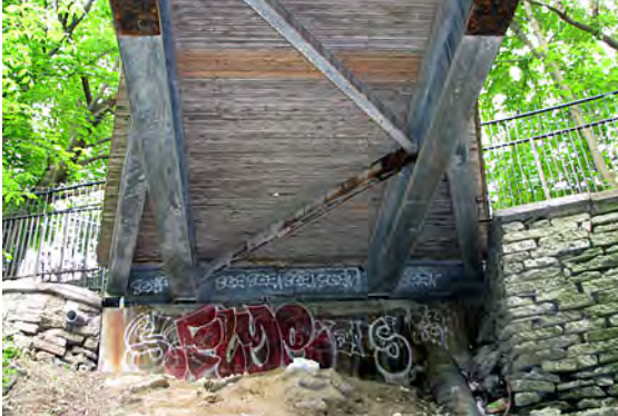
A view south depicts the south concrete abutment with rubble concrete retaining walls.
