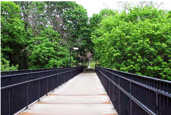
The original open metal handrail system was increased in height during the 2001 rehabilitation of the bridge.
