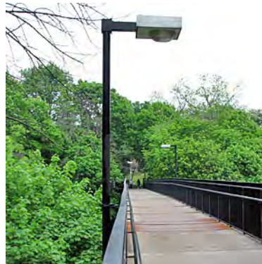
The lighting on the bridge features rectangular light fixtures mounted horizontally on the top of 12-ft. (3.66 m) circular posts.
