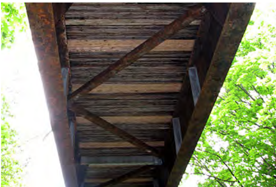
A view of the underside of the bridge shows two girders of weathering steel built up of I-shaped sections, bracing and laminated timber deck.
