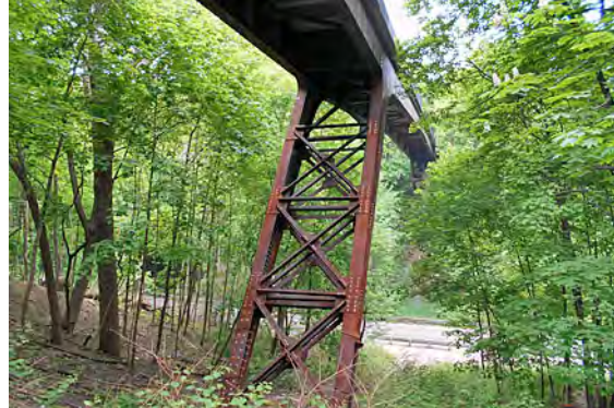
The south pier comprises two inclined girders connected with transverse beams and lateral braces.
