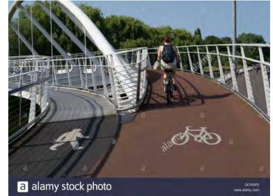
Separate cycling and pedestrian facilities
