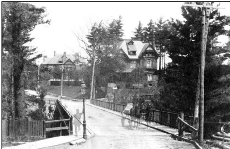
South Glen Road Bridge 1884
