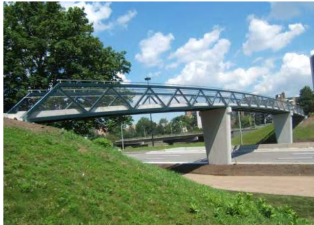
Concrete Steel Truss
