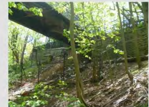
Vegetation around south end of existing bridge (near Bloor Street East)
