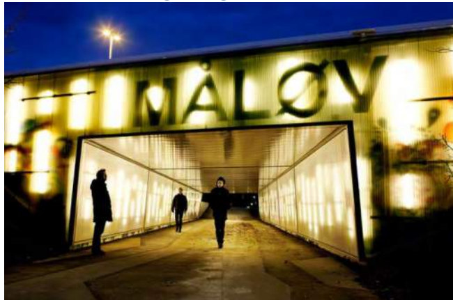
Continuous Lighting in Tunnel
