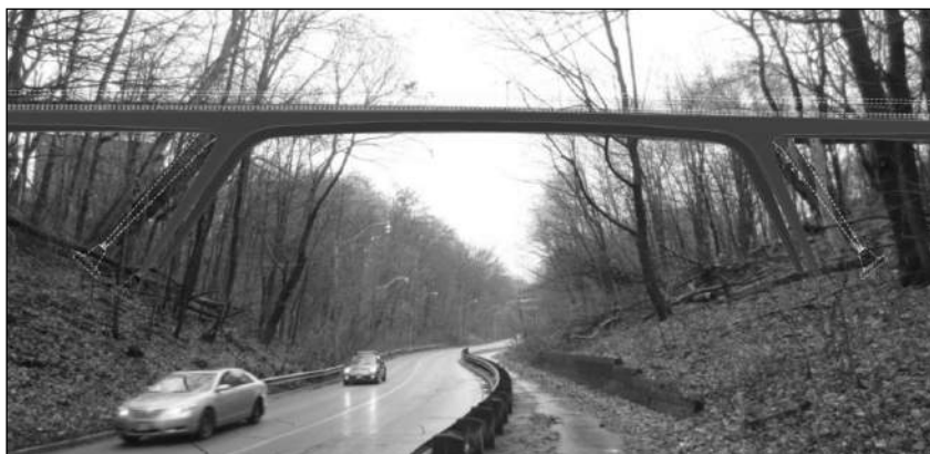
Artist's rendering of recommend structure type: steel girder with inclined steel legs
