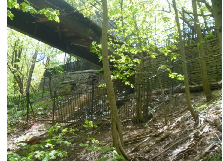
Photograph 3: Vegetation around south end of existing bridge (near Bloor Street East).
