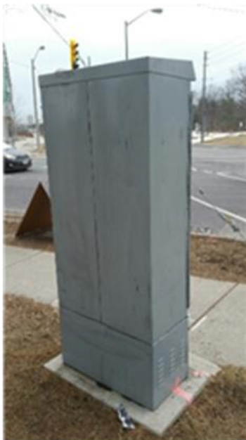
Exhibit 3: Traffic Signal Control Cabinet
