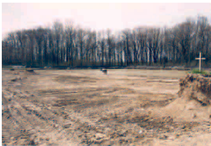
Figure 17 - Example of large scale removal of natural soil during site development
